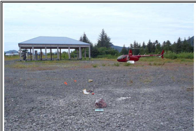
Check Point: 282-1 Photo Date: 7/21/2015 View: South
