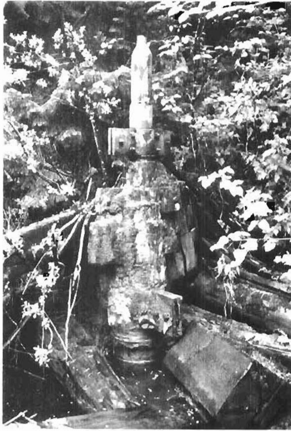
Wellhead of General Petroleum Co.--Sullivan No. 1. This well was drilled near the active Johnston Creek oil seep in 1926-27 to a depth of 2,005 feet and was the first well to test the Sullivan structure. Small bubbles of methane gas issues from around the casing, and a small quantity is emitted from the tubing orifice.
