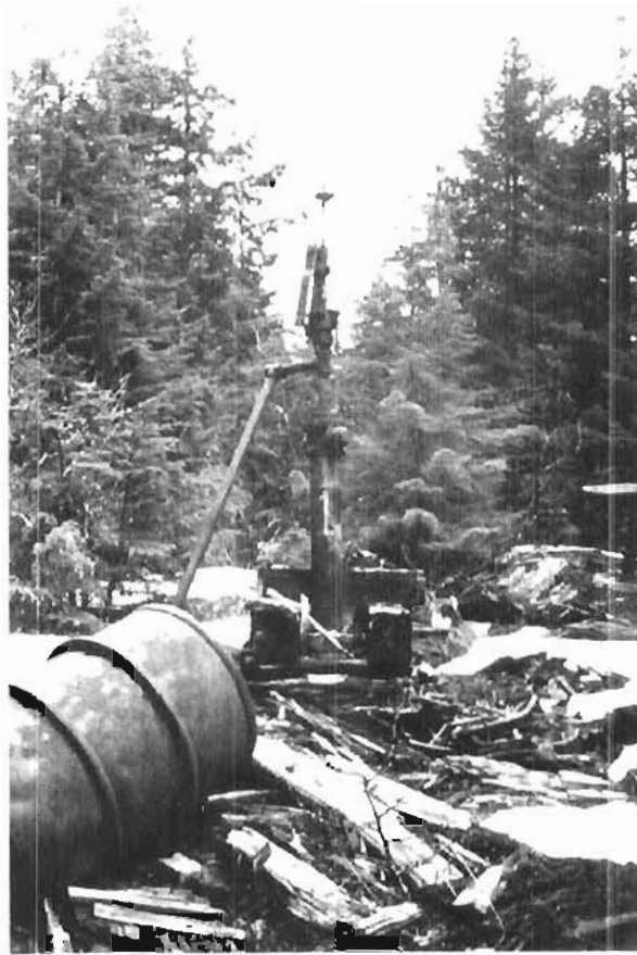
Wellhead of first well drilled in the Katalla Oil Field near the head of Katalla Slough. Katalla No. 1 was drilled in 1902 by the Alaska Steam Coal and Petroleum Syndicate to a depth of 366 feet. On pump it produced oil and considerable gas and helped maintain the Katalla refinery, completed in 1912.
