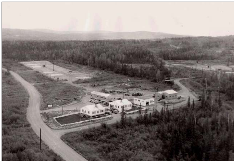
Figure 2. An aerial view of the Fairbanks Permafrost Experiment Station taken in July 1958. The buildings in the photograph are no longer at the site because ground thawing caused settlement and distortion of the buildings. The cleared 'Linell plots' can be seen in the upper right center of the photograph, and an experimental runway can be seen behind the building in the upper left portion of the photo.
