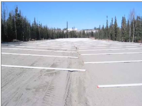
Figure 3. Thermosyphon installation.
