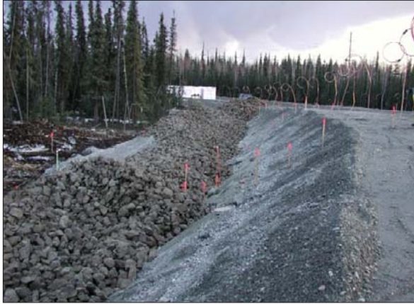
Figure 2. Shoulder installation.
