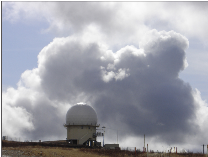
Figure 6. Radar tower at summit of Murphy Dome.
