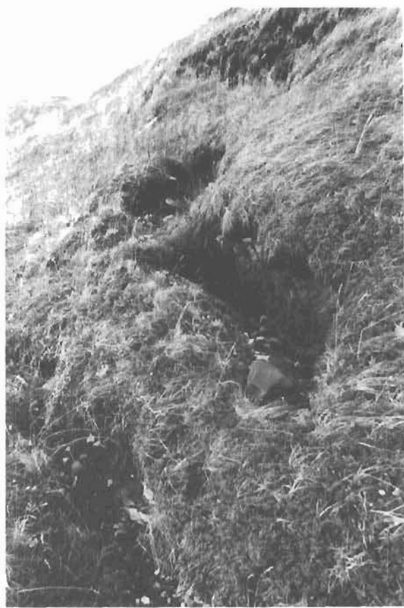
Figure 2. Typical open fissures regarded as active; intermediate slope of Pillar Mountain.
