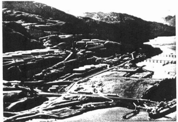
Aerial view of the Alyeska Pipeline Terminal, Valdez, Alaska. Photograph courtesy of Alyeska Pipeline Service Company, 1984.
