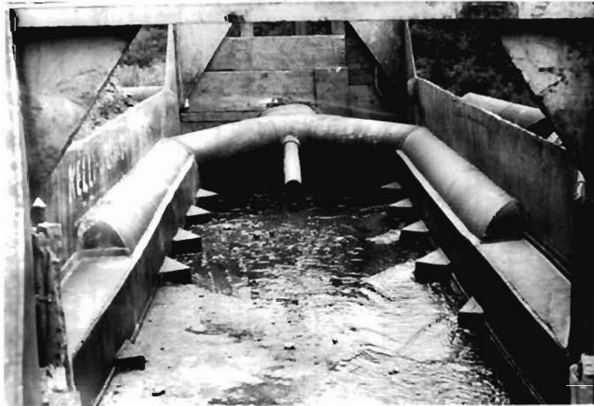
Fig. 1. Box used as a sluice plate by G. W. Carr on Miller Creek.
