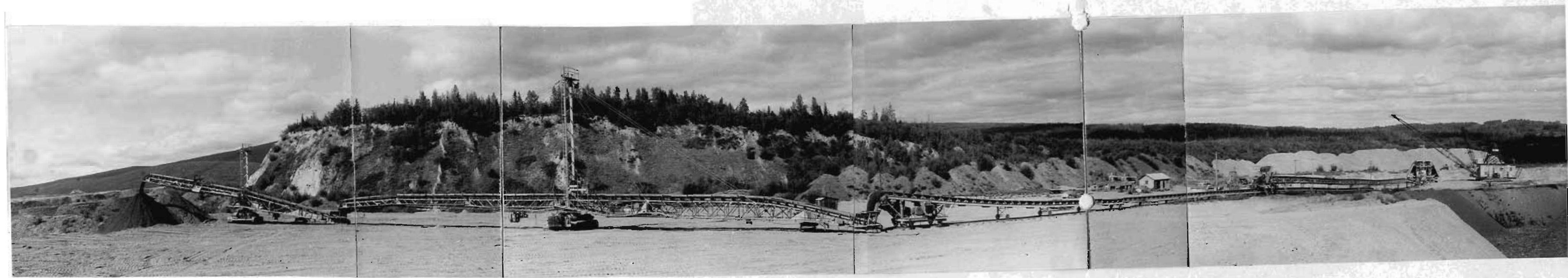
Fig. 12. Dragline and conveyor belt used for stripping barren gravel ahead of Dredge 10 on Gripple Creek.
