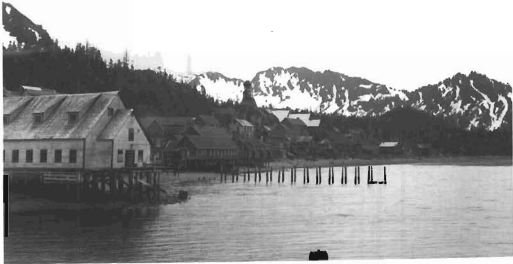
1. View of Latouche from the dock.
