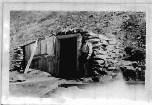
Portal of drift, Mission Creek.
