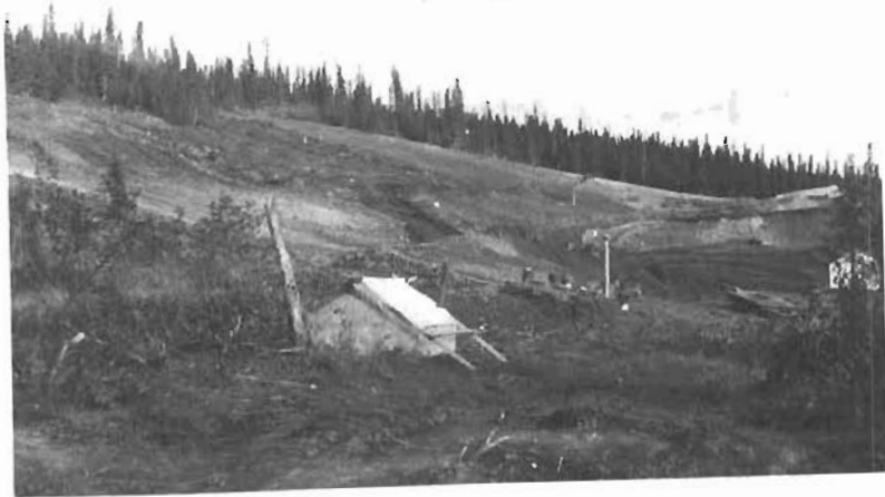
Part of camp and large stripped area.
