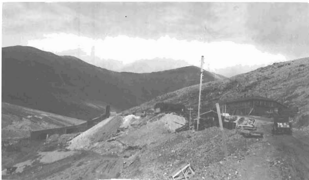
Figure 2. Lost River Mine surface plant.
