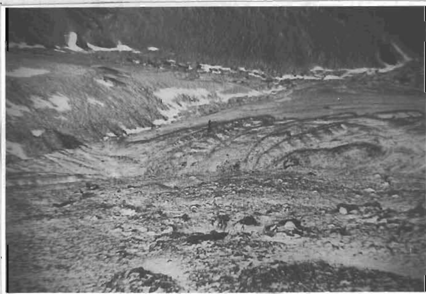
Figure 4. Looking down on prospect showing bulldozer benches as cut in 1951.
