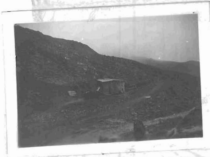
The air compressor which was hauled to the job. Mr. Robert Thorne, Bureau of Mines, in foreground.
