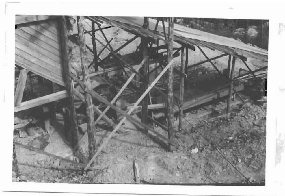
Cully Ore Disintegrator and Straub table in mill.
