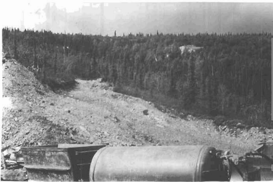
Looking toward Eisenhower adit from new adit.
