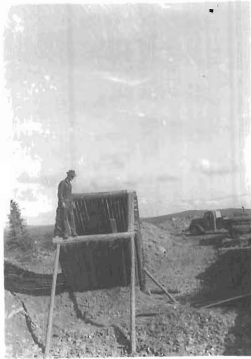
Shaft timbers in place in Trench 3.
