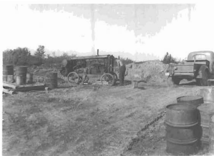
Compressor used for shaft sinking.
