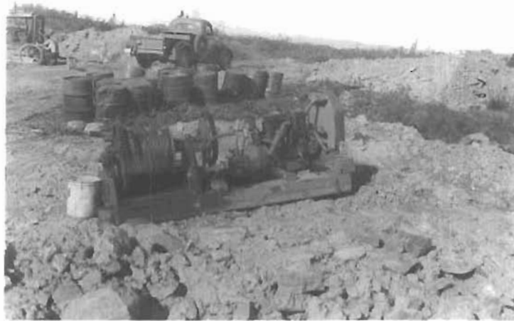
Hoist and engine used for shaft sinking.
