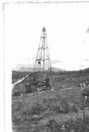
Drilling operation ahead of dredge
