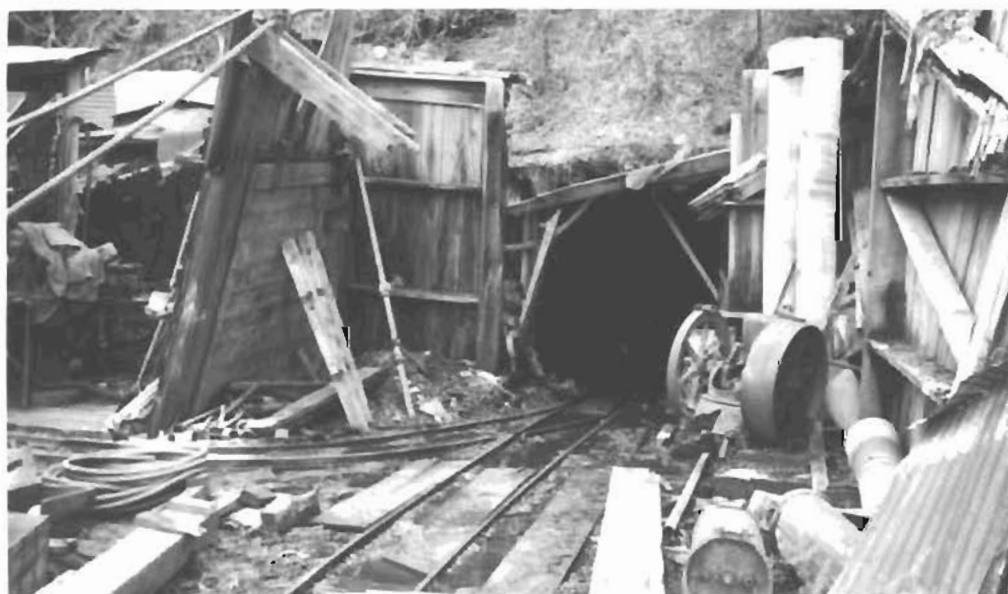
Figure 7. No. 9 Level Portal.
