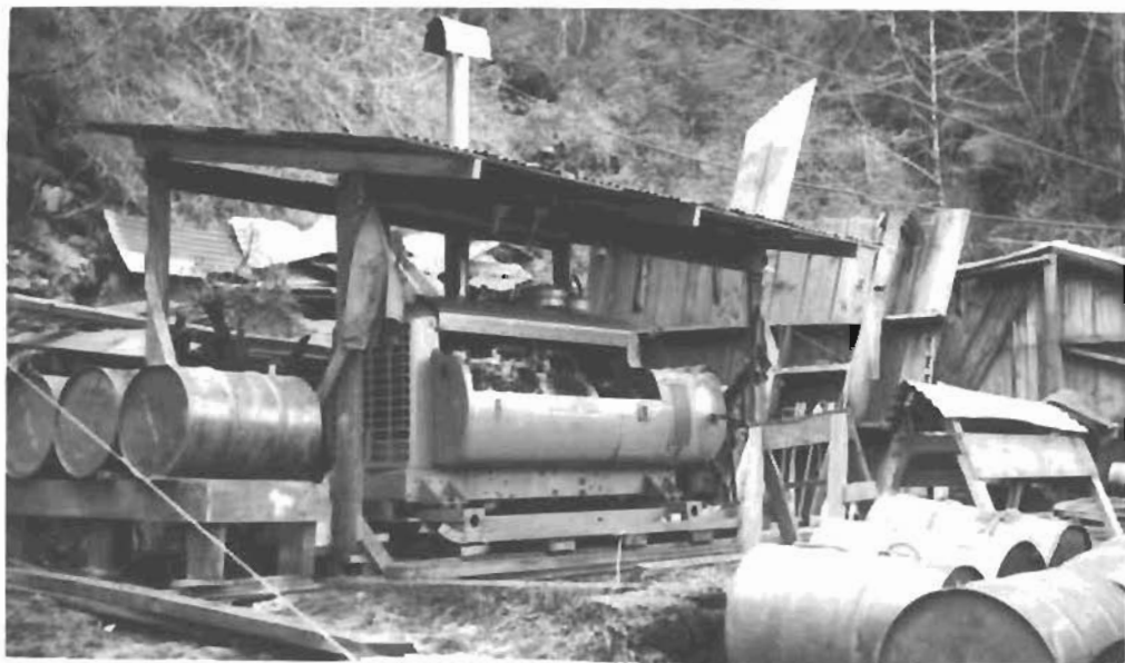
Figure 6. Compressor used by Alaska Copper Corp. at portal of No. 9 Level.
