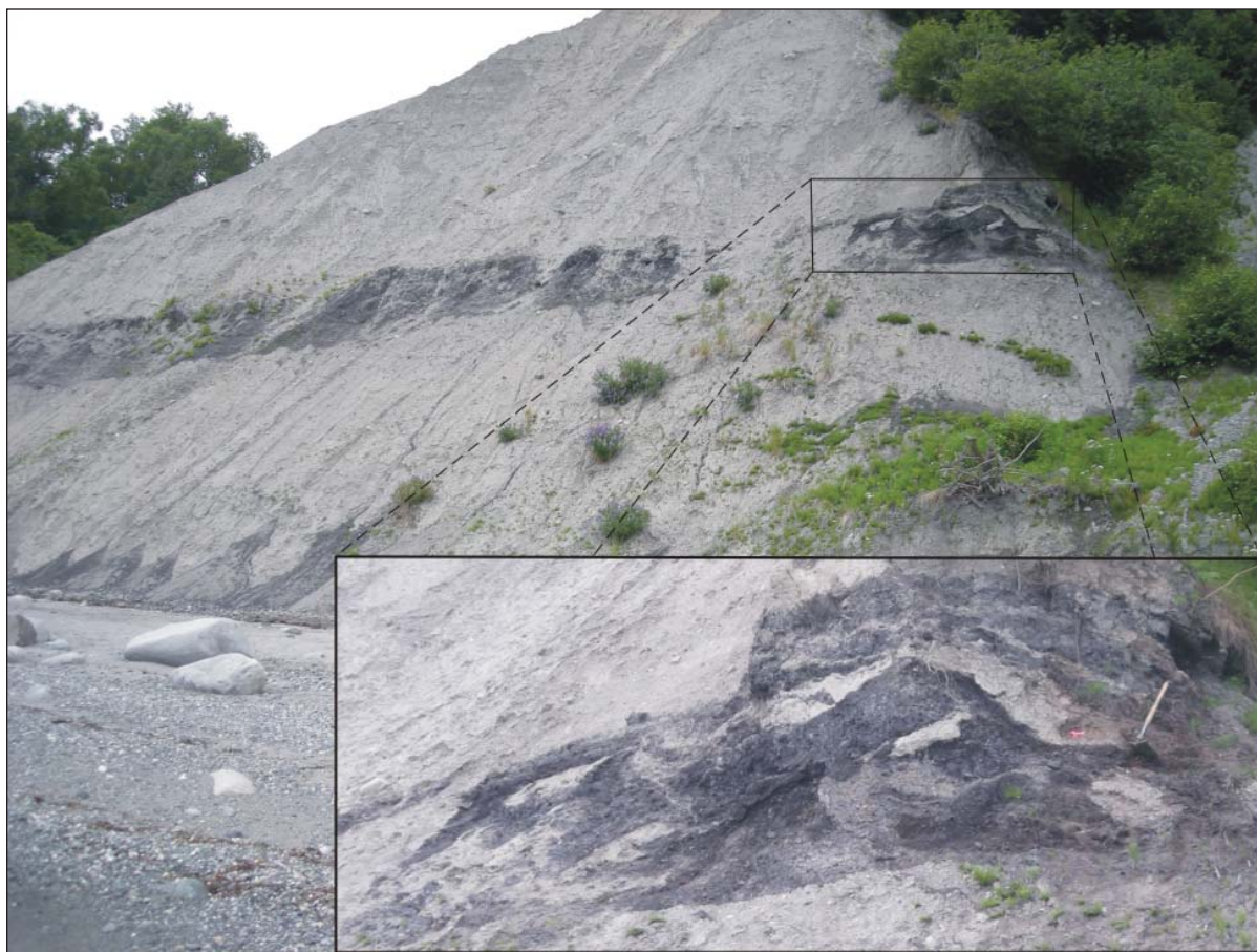
Figure 5. Prominent coal bed exposed in coastal bluff between ~150 and ~230 m northeast of pipeline centerline. Inset shows intensely fractured, pulverized, and distorted allochthonous coal mixed with pebble diamicton. Shovel handle is 0.5 m long. Photographs taken 07/15/08.
