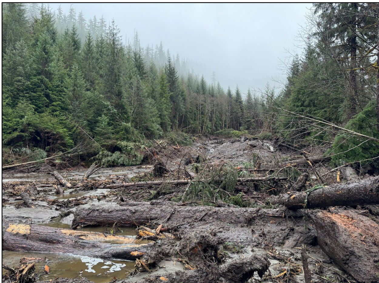
Figure 6. Toe of the Middle Ridge Road landslide where it covers the road (photo looking south by Barrett Salisbury, November 24, 2023).
