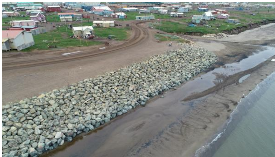
Oblique imagery of the rock revetment protection in Wainwright, Alaska (DGGs, 2023)
