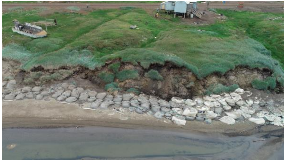
Oblique imagery of sandbag semi-protection in Wainwright, Alaska (DGGS, 2023)
