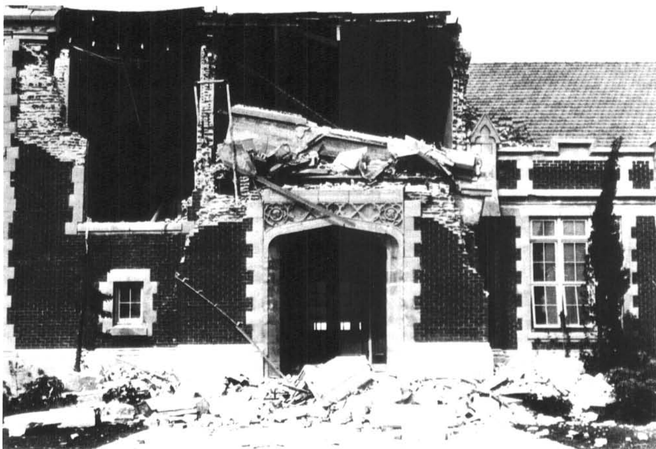
Figure 14. John Muir School, Long Beach, California, damaged by the March 10, 1933, earthquake (Richter magnitude 6.3). Photograph by W.L. Huber.
