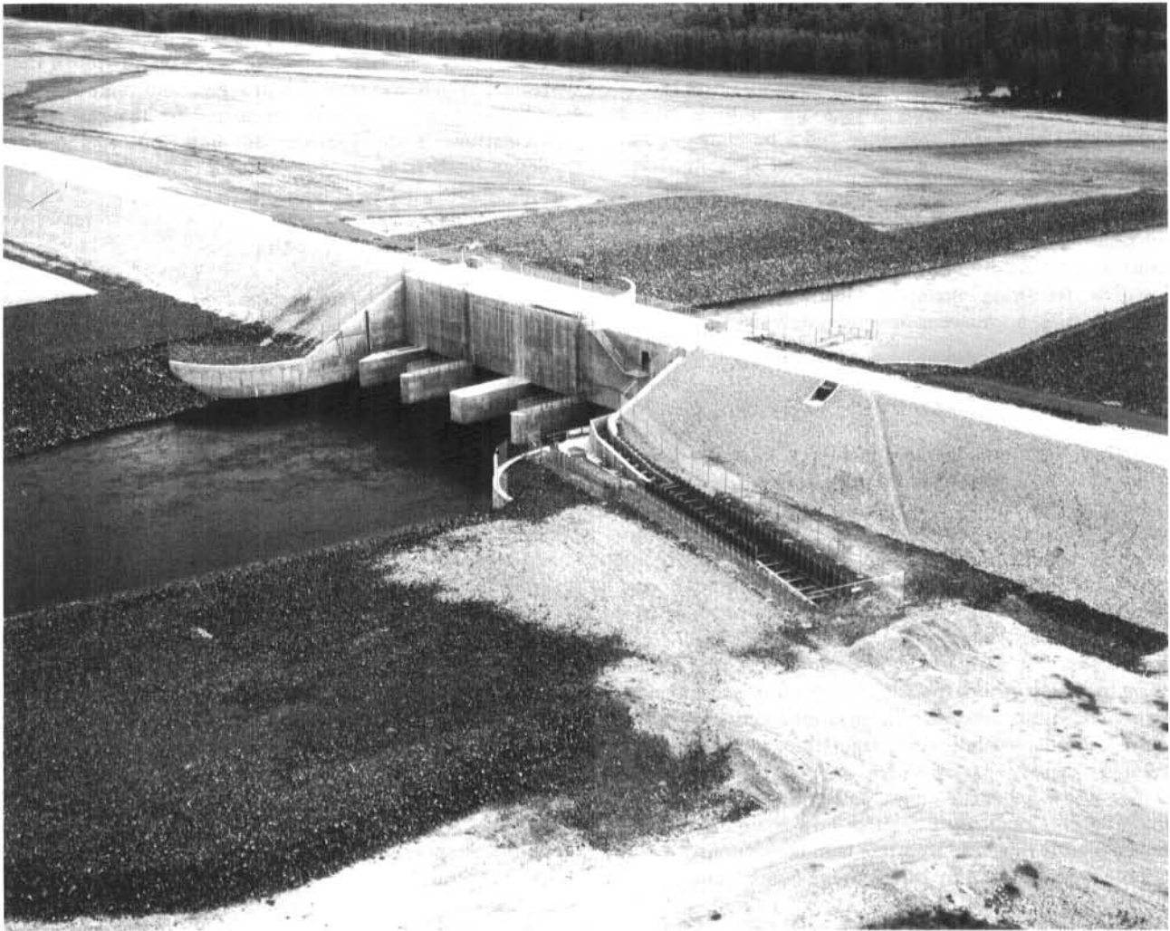
Figure 11. Floodgate in the Chena Lakes Flood Control project, about 20 mi east of Fairbanks. The structure limits water flow to 12,000 \text{ ft}^3/\text{sec} , which is less than one-fifth the amount that flooded Fairbanks in 1967. Photograph by U.S. Army Corps of Engineers.
