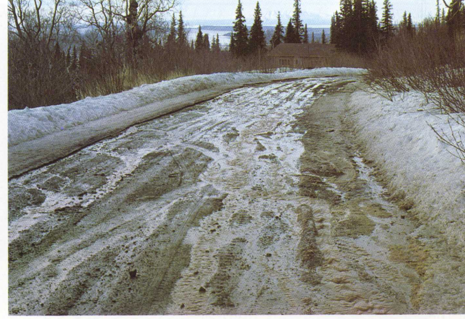
Figure 3c. -- Erosion of road by melt water during the spring (Spain Drive near Potter Creek, April 1980).
