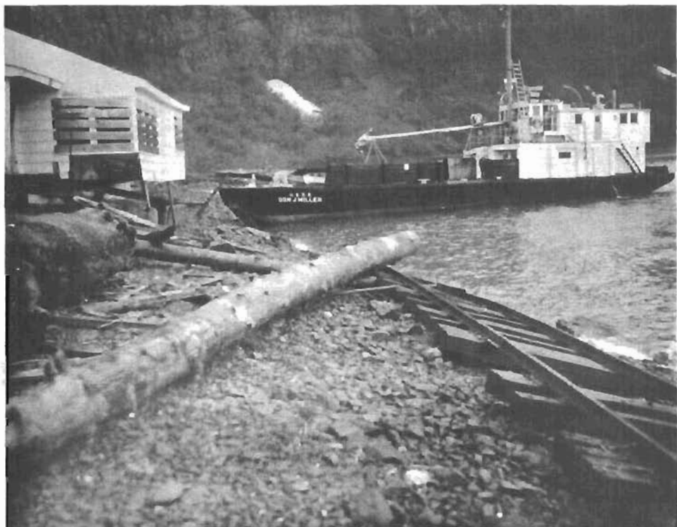
Figure 15. Slide scarp in terminal moraine-outwash-delta complex at the head of Passage Canal. The submarine slide carried away a portion of the railroad spur in the right foreground and partially undermined the abandoned house shown at the left. Water depth beneath the stern of the boat is 63 feet, indicating a submarine slope of 32 degrees. Prior to the earthquake the tidal mud flats extended 75 feet out from shore at this point. Photo by G Dallas Hanna.
