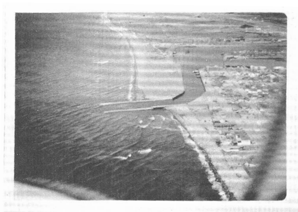
Figure 28.--The Snake River jetties showing accumulation of sediment on the west side and erosion on the east. Looking west with the town of Nome in the foreground.
