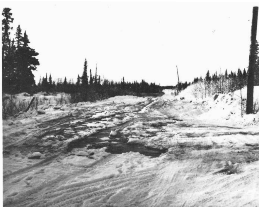
Figure 16.-- Summer drainage and winter icing at Patrick Road and upper DeArmoun Road. Year-round ground-water seepage from a nearby slope has caused a buildup of ice in the roadside ditch during winter months. This icing in December 1971 created impassable road conditions for several weeks. Excess water flowed over the icing, infiltrated the snow cover, and then seeped over the frozen ground into nearby yards.
