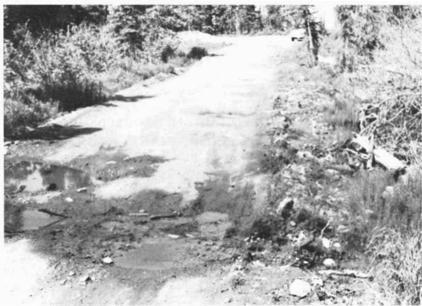
Figure 15.-- Ground-water seepage crossing road in upper O'Malley area.
