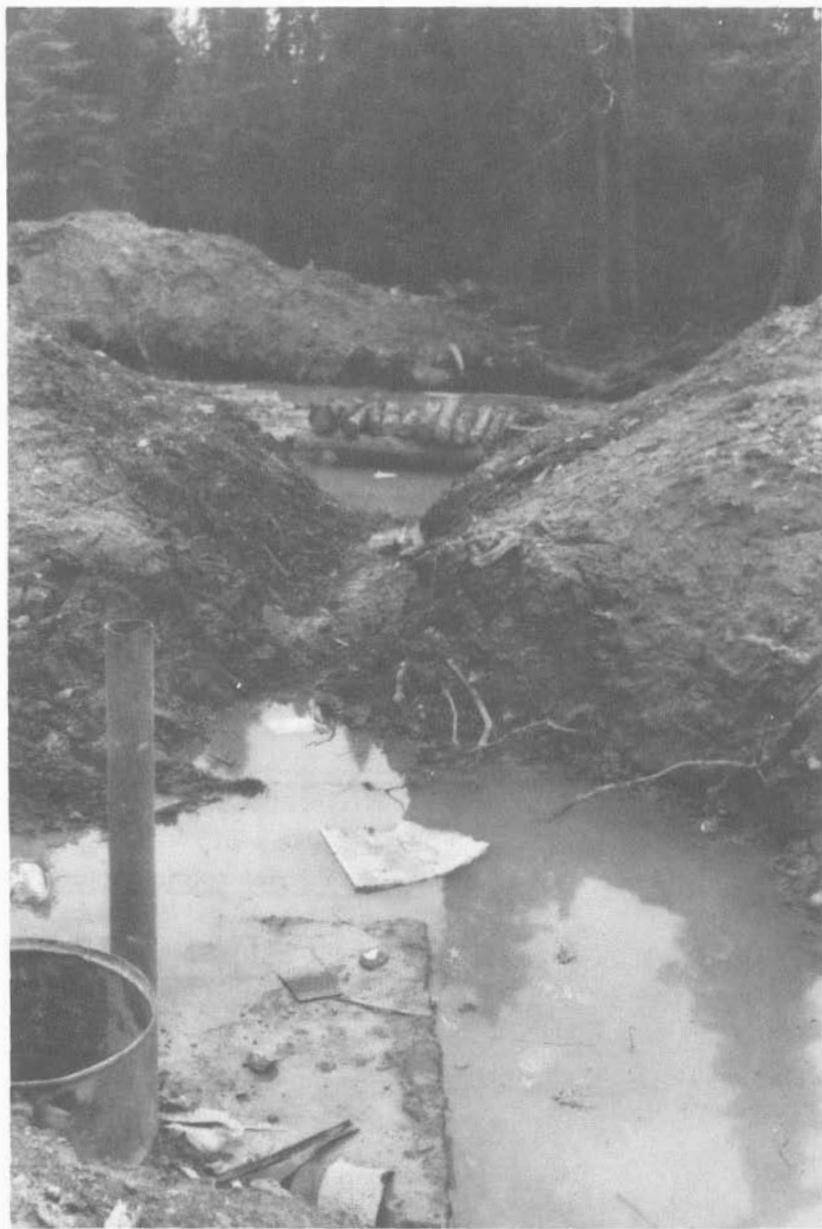
Figure 27.-- Cesspool cribbing floating in shallow ground water.
