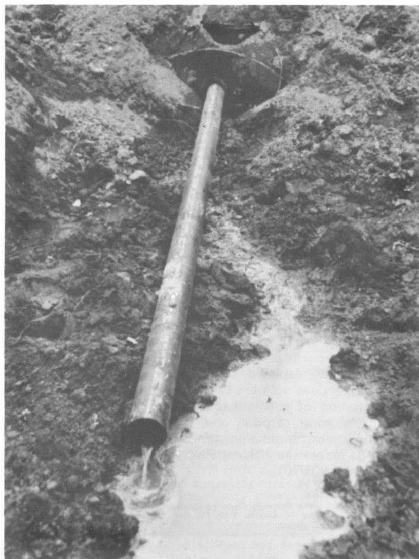
Figure 24.-- Ground water flowing through partly buried septic tank.
