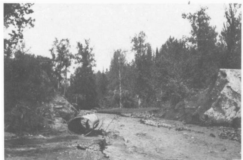
Figure 19.-- Washout of Old Seward Highway roadbed by 1964 flood on Rabbit Creek.
