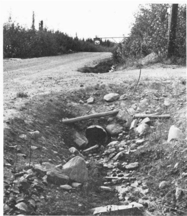
Figure 16.-- Summer drainage and winter icing at Patrick Road and upper DeArmoun Road. Year-round ground-water seepage from a nearby slope has caused a buildup of ice in the roadside ditch during winter months. This icing in December 1971 created impassable road conditions for several weeks. Excess water flowed over the icing, infiltrated the snow cover, and then seeped over the frozen ground into nearby yards.
