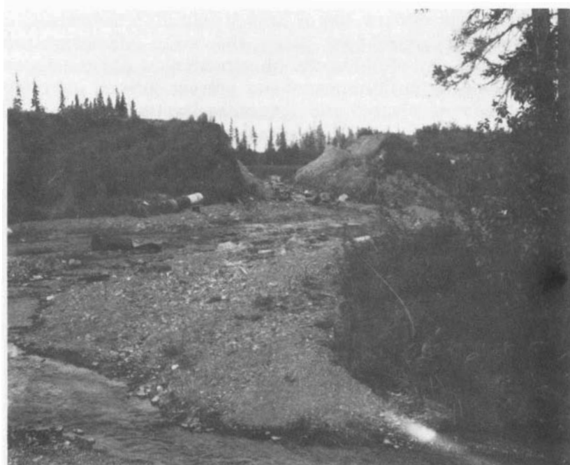
Figure 20.-- 'Lake of the Hills' earth dam after failure in 1972.
