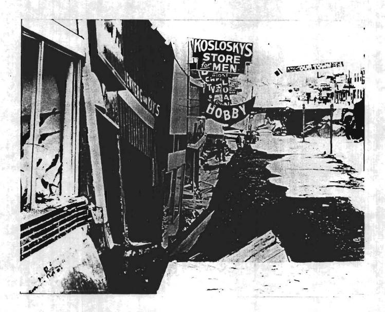
Figure 1. Fourth Avenue landslide scarp immediately after March 27, 1964
