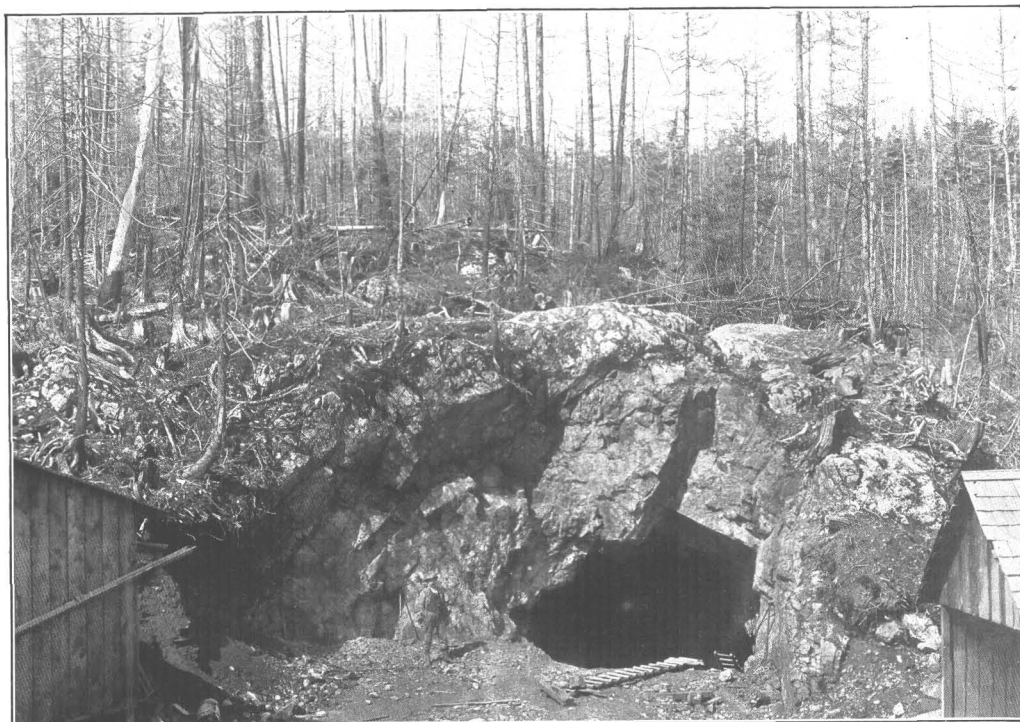
B. ENTRANCE TO SLOPE AND SURFACE CAPPING OF ORE BODY AT RUSH & BROWN MINE.
