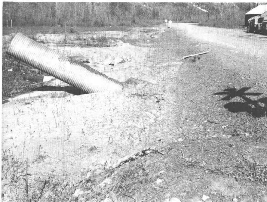
119.—Three-foot-diameter culvert cantilevered upward by sinking of the highway fill just north of the grade crossing at mile 62.9.
