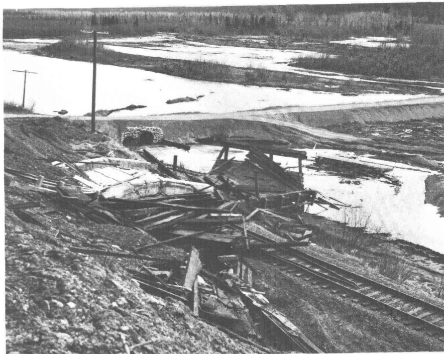
87.—The concrete deck of a highway overpass at Snow River delta that collapsed onto the railroad.
