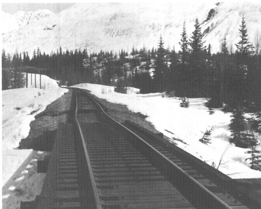
102.—View north over bridge 41.6, where 18 feet of the approach fill was lowered about 1.5 feet. Photograph by The Alaska Railroad.
