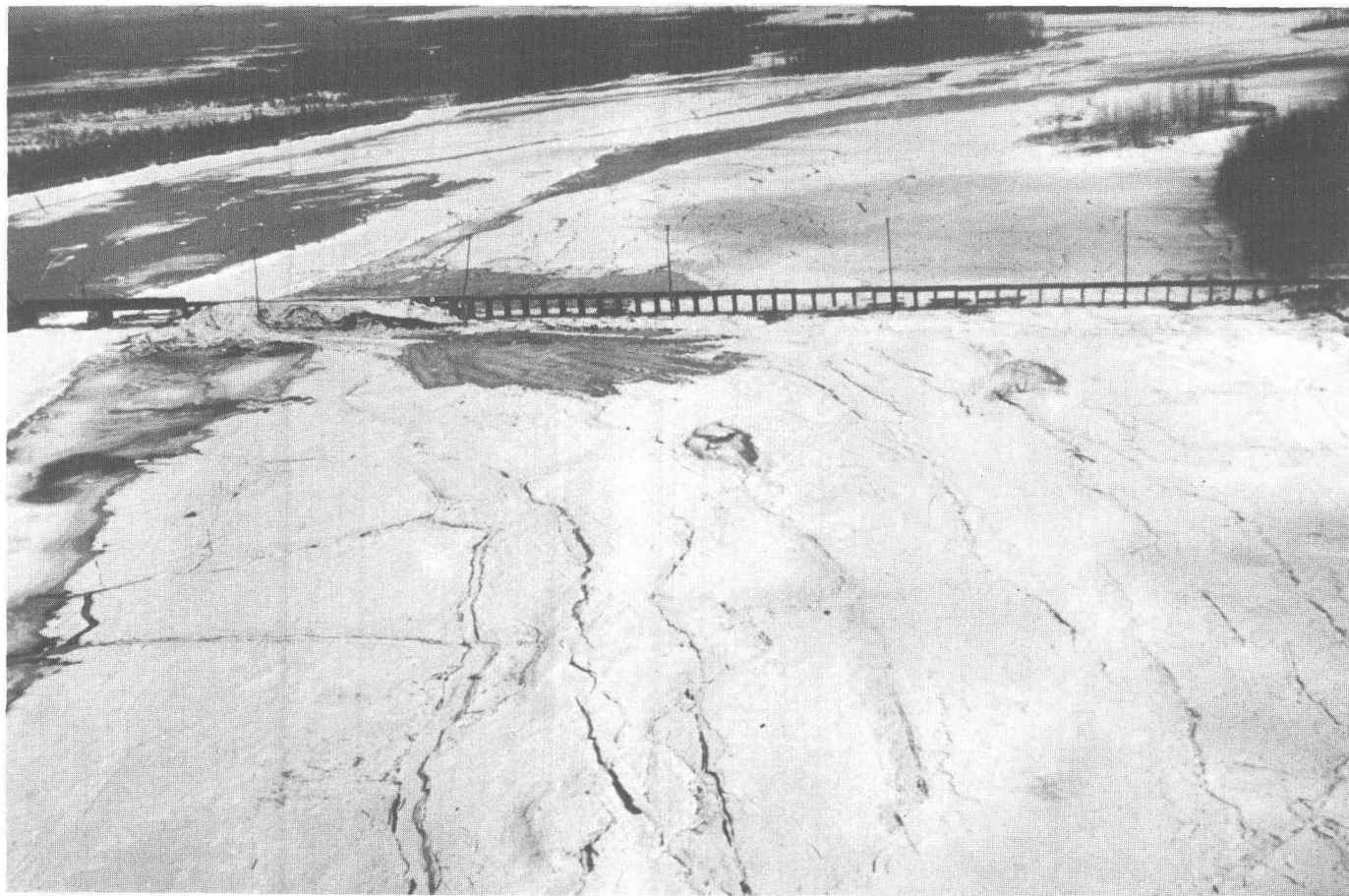
139.—Cracks in the active flood-plain sediments at the south end of bridge 147.5 at Matanuska River. An earth fill has been bulldozed in to replace a section of trestle in which cracks sheared wood piles at the ground and offset the trestle.
