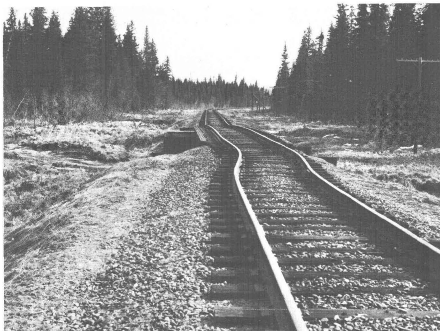
83.—Bridge 15.6, a 45-foot wood trestle on the inactive floodplain of Snow River, showing long, horizontally offset embankments. A, View north; B, view south.
