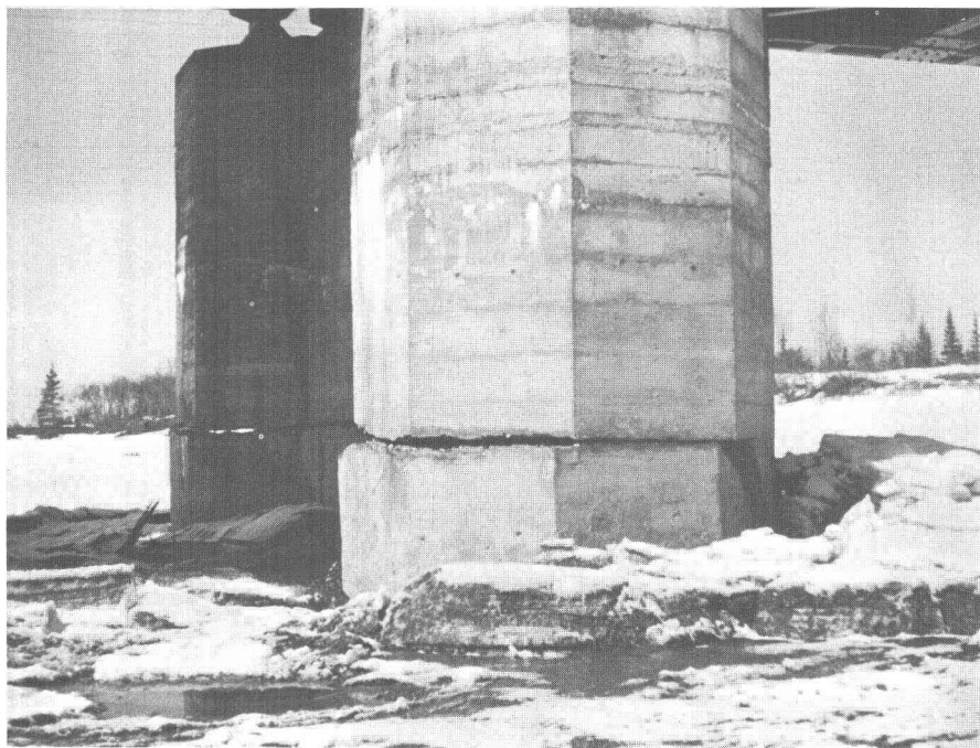
138.—Shearing at a pour joint of a concrete pier at bridge 147.1, Knik River.
