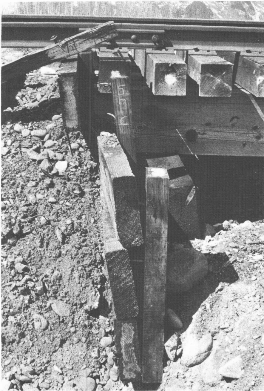
105.—The stringers of bridge 59.6 driven into and through the bulkhead planks.
