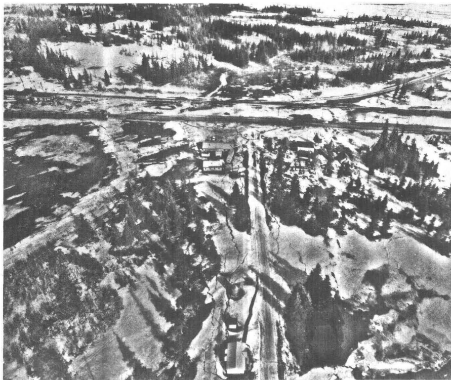
49.—Ground cracks generated by an embankment in Portage. Note dark areas flooded by ground water. Photograph by U.S. Army.
