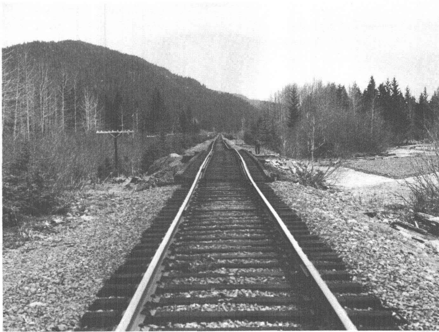
79.—View north over arched and compressed bridge 4.8. Sags of about 2 feet and horizontal displacement of about 1 foot can be seen in the roadbed to the north.
