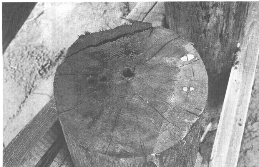
41.—Two impact holes made by a drift pin in the pile cap as the deck of the bridge was alternately raised and lowered onto the piles (see also figs. 13, 95). Stream channel is to the right.
