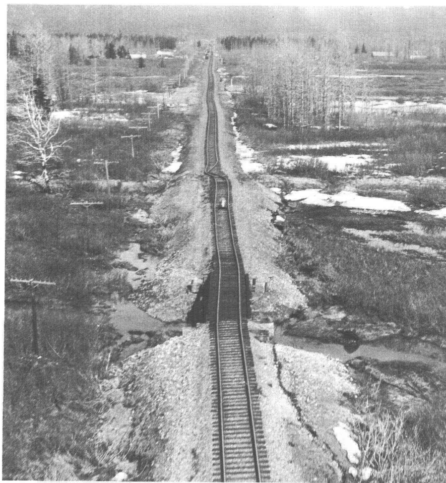
116.—Broken and laterally displaced embankment north of bridge 62.3. Photograph by The Alaska Railroad.
