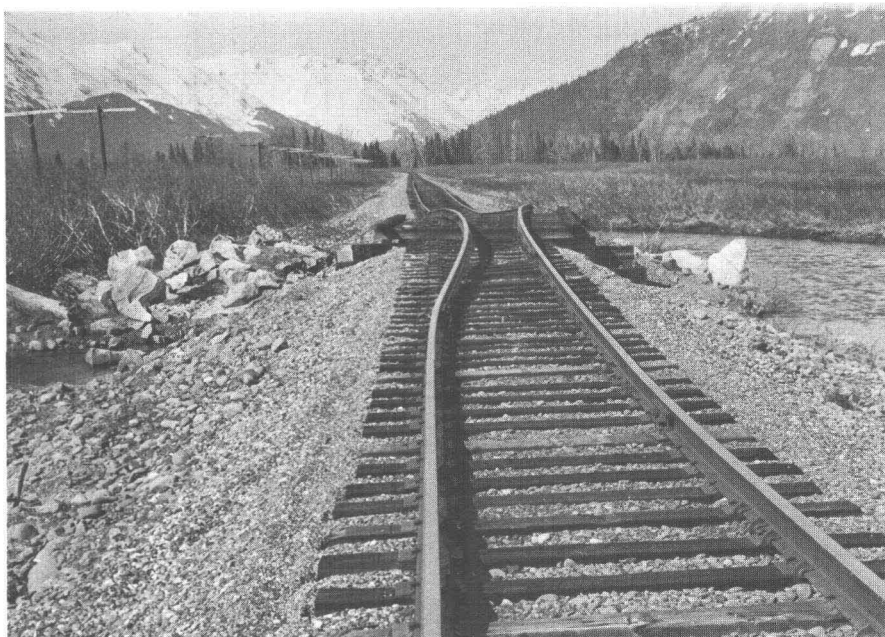
108.—View north over bridge 61.5 on the inactive flood plain of Portage Creek. The bridge was compressed and arched, and the rails pulled free of the fish plates. The north approach shifted to the right toward a small slough, and the south embankment shifted toward the topographically lower active flood plain of the adjacent creek, skewing the bridge 18 inches horizontally (see fig. 56).
