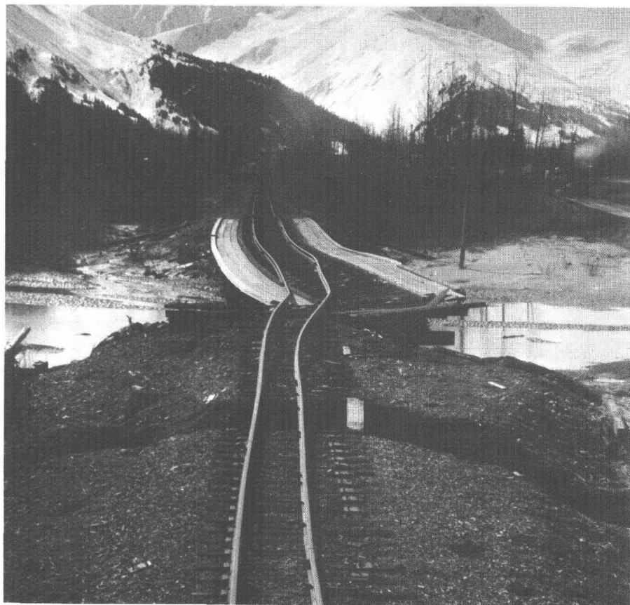
18.—View to the south of bridge 63.0. Compression, which deflected the deck 8 feet to the east in a sharp kink, broke the stringers. A wide tension fracture in the foreground broke the embankment; it shifted to the right at the fracture and skewed the bridge.
