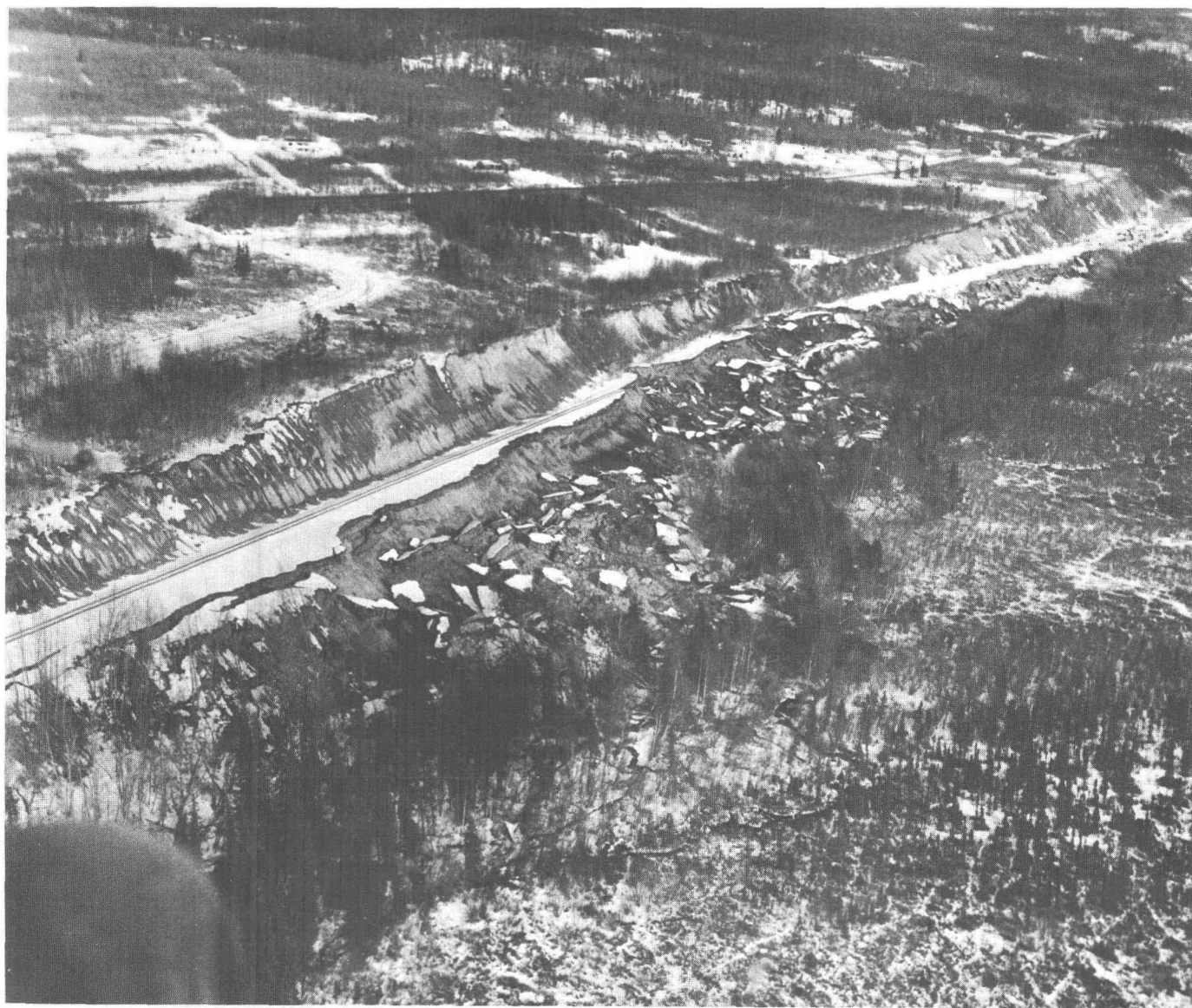
65.—View of Potter Hill slides. Note the overthrusts in the low-lying tidal flat in the foreground, and dark strata of water-saturated sediments in the slide scarps. Photograph by The Alaska Railroad.
