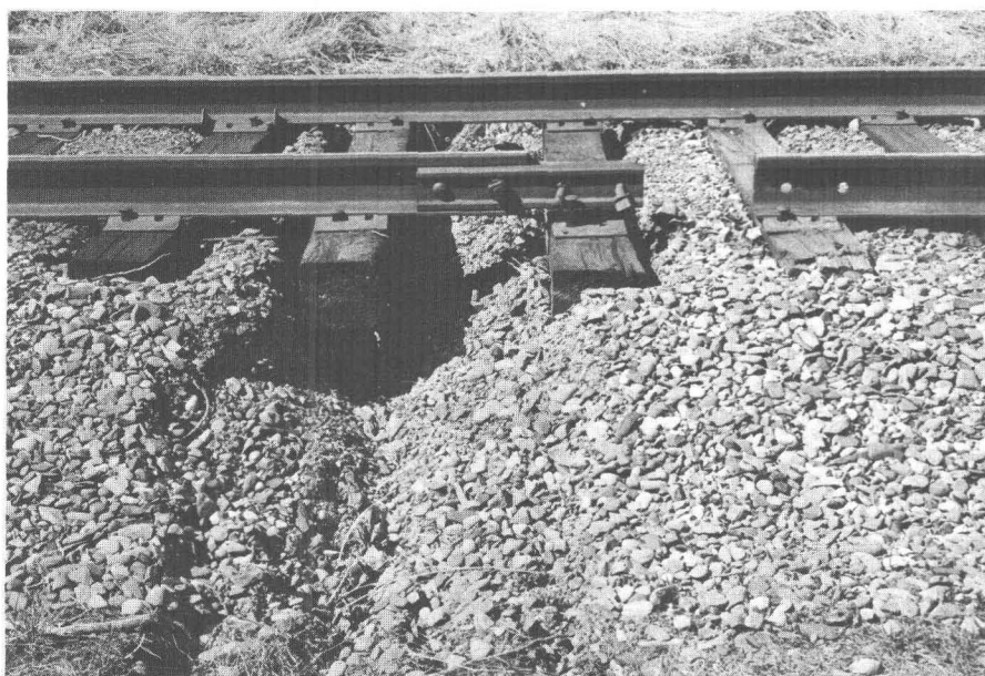
118.—Tension fracture in the roadbed and a 2-foot pull-apart in the rail at about mile 61.9 caused by spreading of the underlying flood-plain sediments (see pl. 3).
