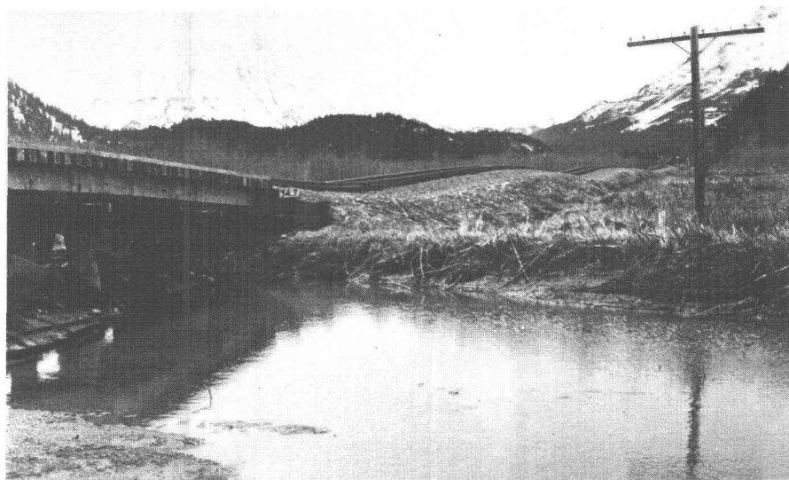
96.—Local settling of the railroad embankment between bridges 34.7 (foreground) and 34.5 on Hunter Flats.
