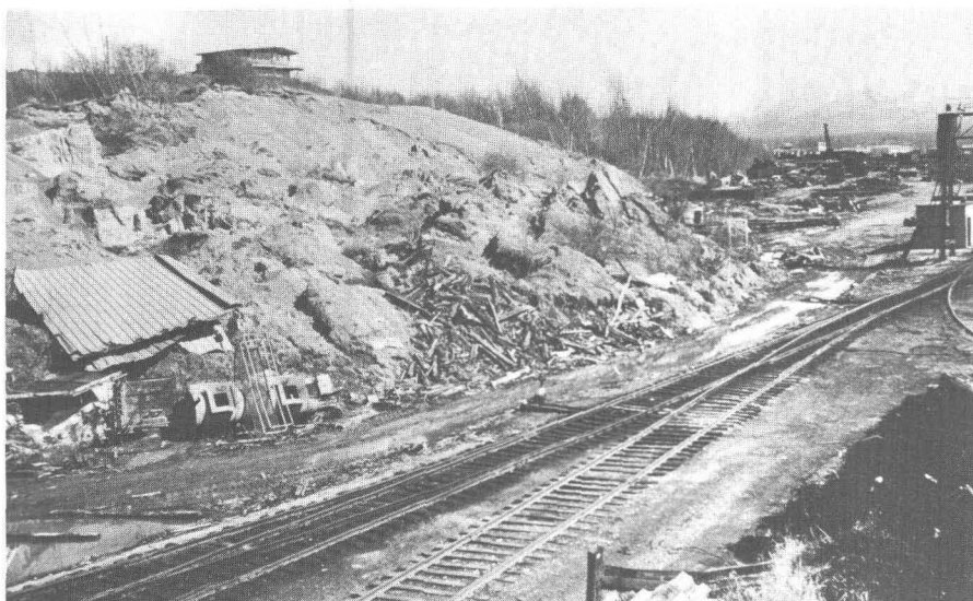
135.—The toe of Government Hill slide that overran an on-track storage building and some rolling stock on the north side of Ship Creek valley
