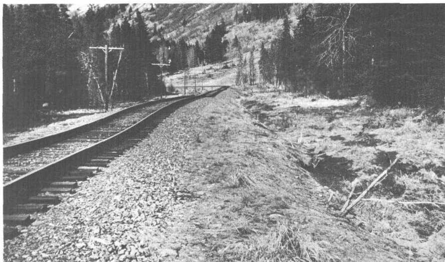
84.—Mounds of sand and gravel ejected with ground water coincident with local dips in the embankment (foreground and middle ground).
