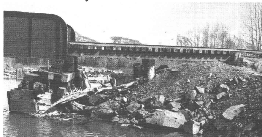
Streambanks moved closer together, driving wood stringers into the central span and about 1 foot past the bulkhead piles. The bulkhead was rotated and driven into the fill, and the guard timber was shoved over the top of the bulkhead. The rails were pulled free of the ties on the approach fill. The piles between the wood spans were shifted 22 inches to the left of the pile cap. Light-colored pile in foreground from older bridge
