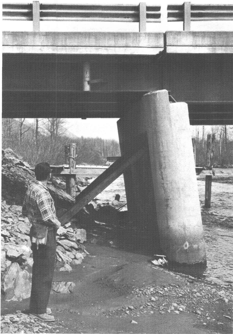
6.—The pier of a highway bridge at Resurrection River that was rotated as its base was carried toward the channel while its top was restrained by the deep central steel deck beam. A crack that formed in the pier is visible just above the water.
