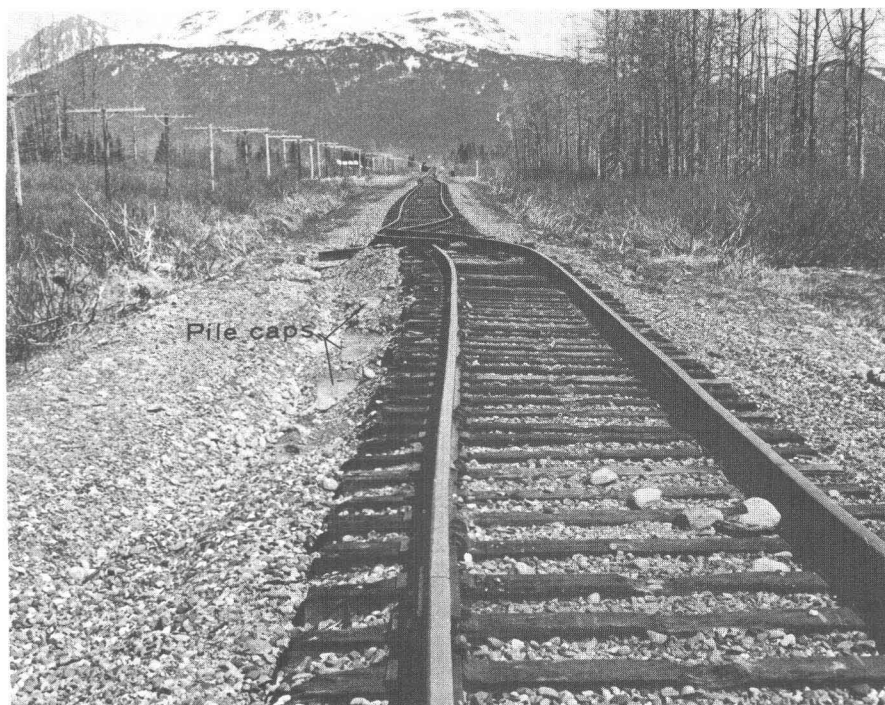
60.—Lateral offsetting and compression at the end of filled-over bridge (looking north toward bridge 62.3). Note the ends of pile caps exposed to left of the ties.
