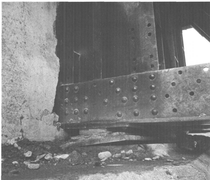
37.—Damage to Twentymile River bridge. Left: Concrete abutment broken away after earthquake to relieve pressure on spans. Note tilted bearing shoe and missing sheared-off anchor bolt. Right: North abutment backwall broken by thrust of steel deck.
