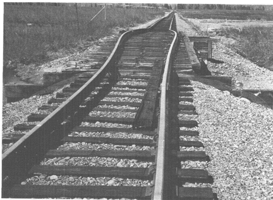
107.—View north over bridge 61.3 on the inactive flood plain of Placer River. The bridge was compressed and arched, and, as shown by the freshly exposed unweathered wood on the bulkhead, the embankment settled at the bulkheads. Approximately 200 feet of the embankment north of the bridge shifted to the left.
