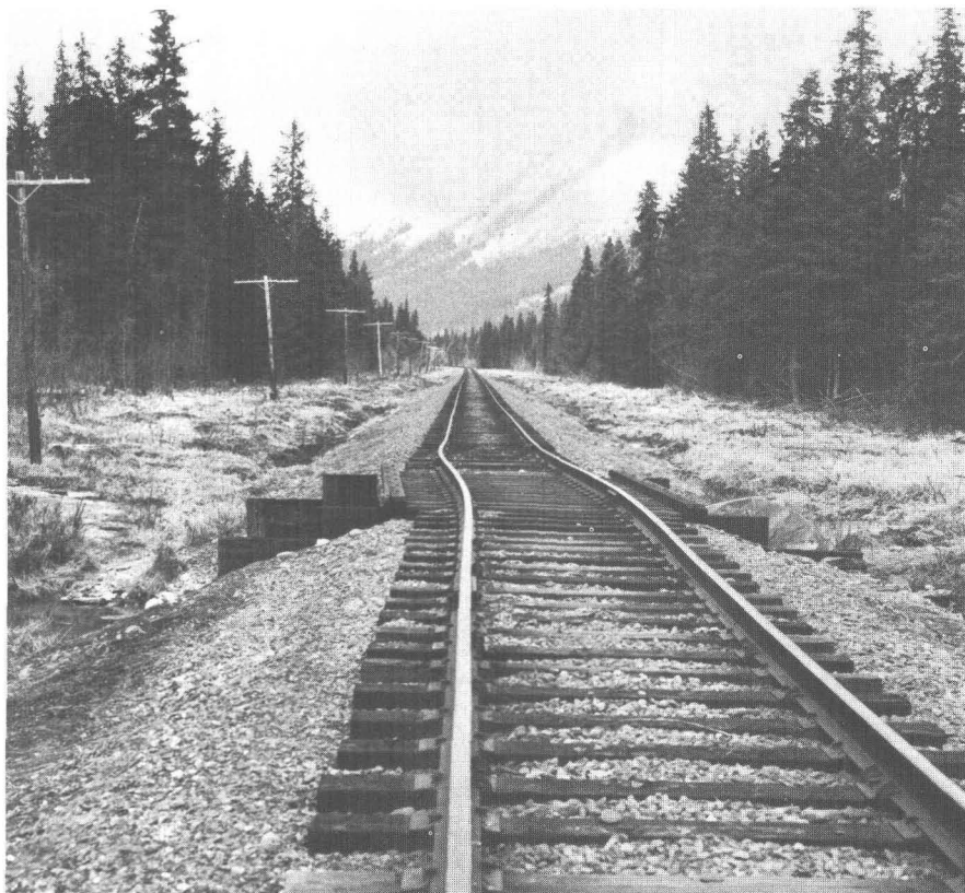
82.—View north over bridge 15.2 on the inactive floodplain terrace of Snow River. Approximately 950 feet of the embankment north of the bridge shifted about 1\frac{1}{2} feet to the west toward an abandoned stream channel 220 to 230 feet to the west, in the tree-covered area.
