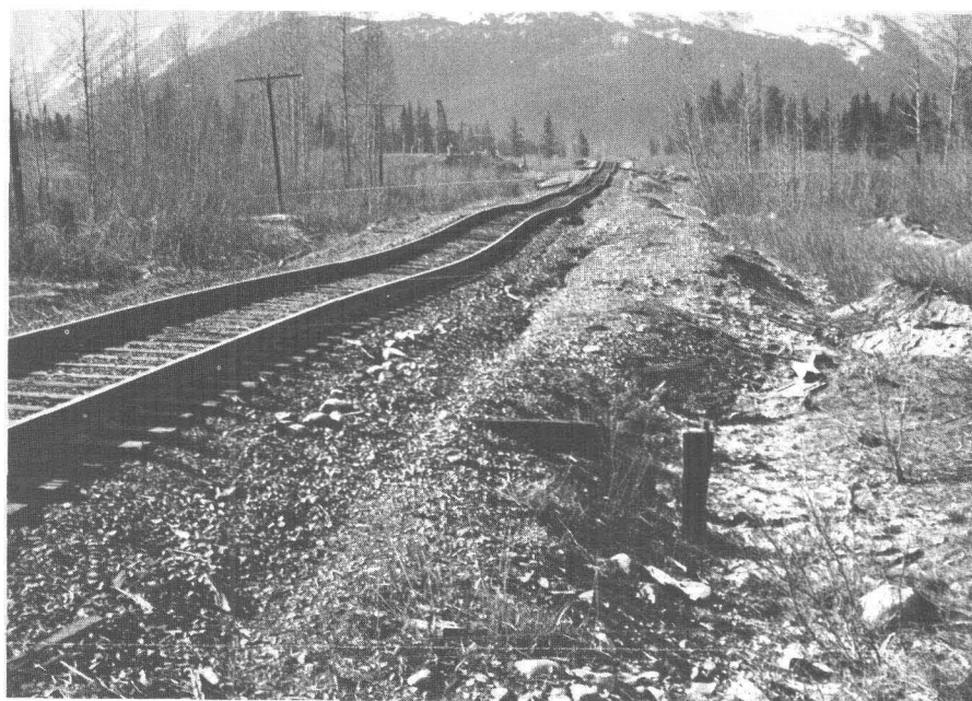
120.—Irregular settlement of the railroad embankment between the highway grade crossing at mile 62.9 and bridge 63.0 (see pl. 3).
