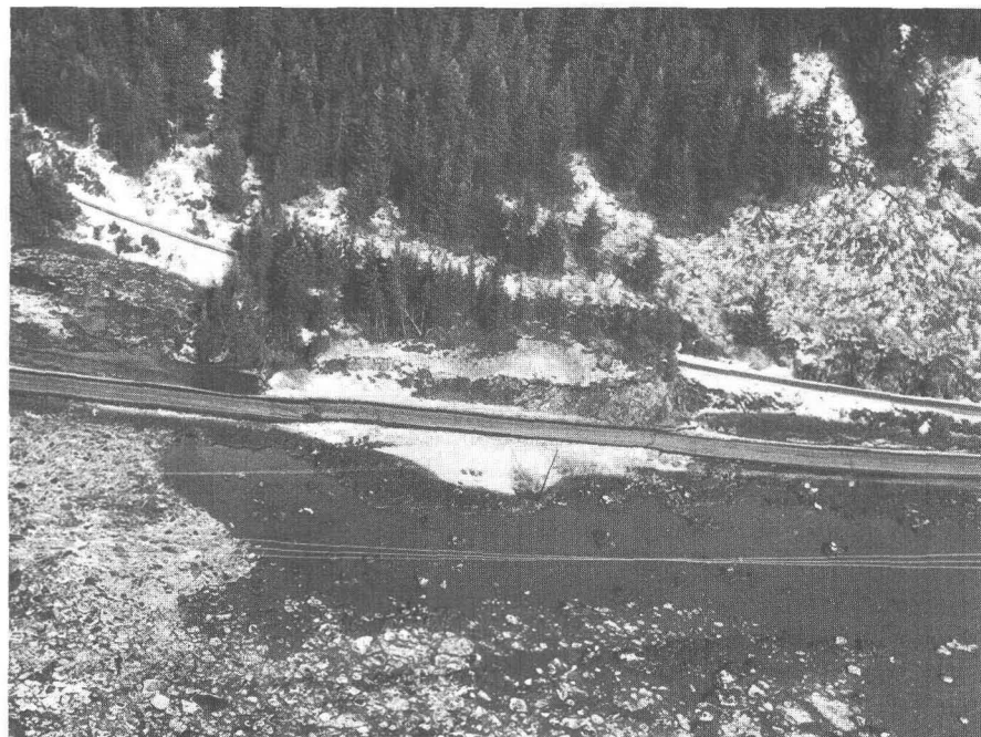
125.—Highway embankment along the north shore of Turnagain Arm that settled abruptly on tidal sediments adjacent to a bedrock promontory. Similar settlement occurred on the railroad embankment. Embankments on tidal sediments also were shifted toward the arm and offset horizontally.
