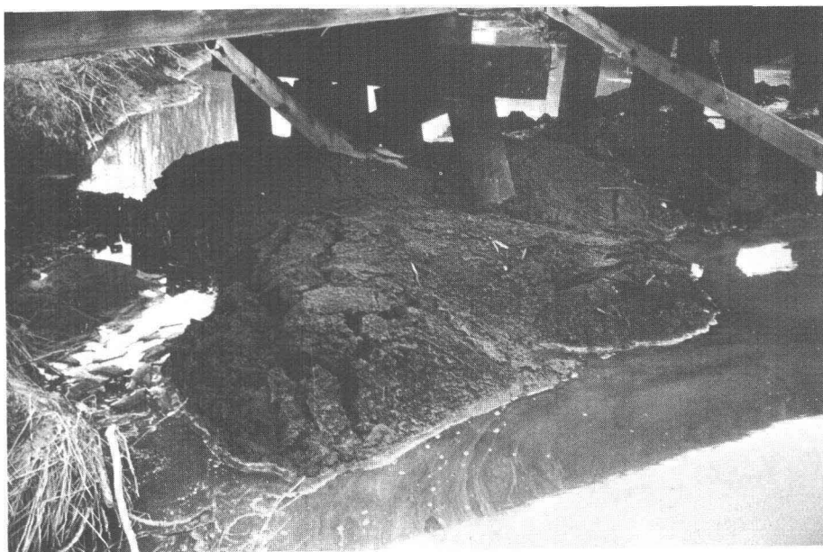
17.—Mounds of sand ejected with ground water from cracks in the floor of the stream at bridge 34.7 on Hunter Flats.
