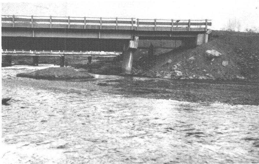
30.—Looking southeast toward highway bridge (No. 596) at Resurrection River. Streamward movement of the foundation materials compressed the deck, breaking the abutment backwall, and carried the abutments and bases of the piers toward the channel. Being restrained at the top, the pier was broken at the ground line. Similar damage occurred at the other end of the bridge.
