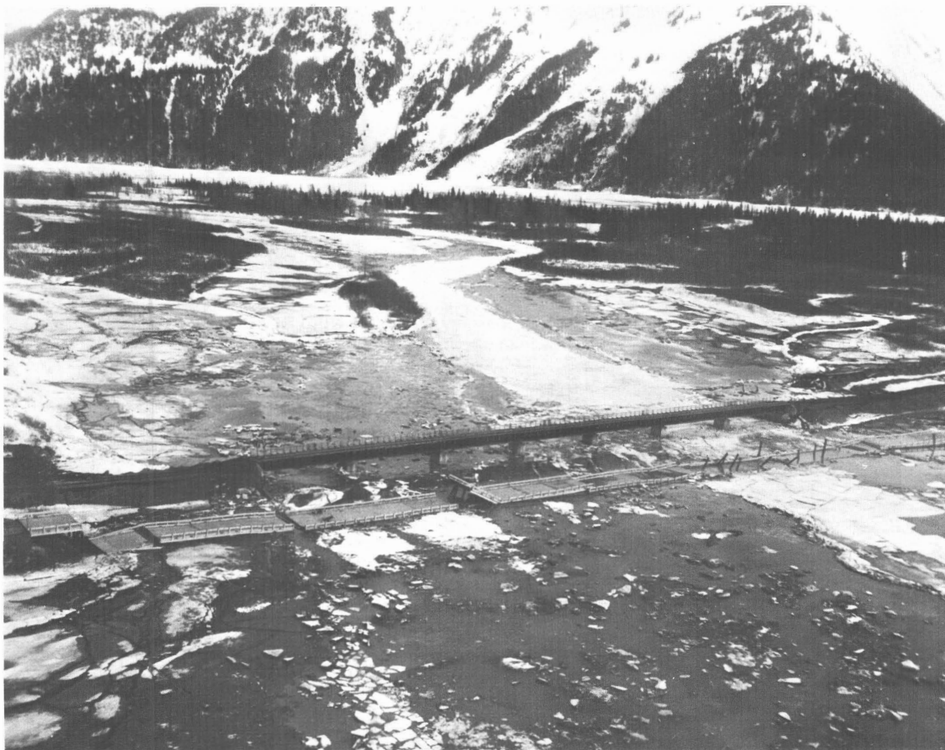
35.—Railroad bridge (64.7) and highway bridge at Twentymile River, Portage. All concrete deck sections of the highway bridge except one were knocked from their piles, and some piles were driven through the concrete. The railroad bridge was compressed and some of its piers shifted (see fig. 36). Note the severe cracking in the embankments, flood-plain, and tidal sediments (see pl. 3). Photograph by Arthur Kennedy, U.S. Forest Service, Anchorage.
