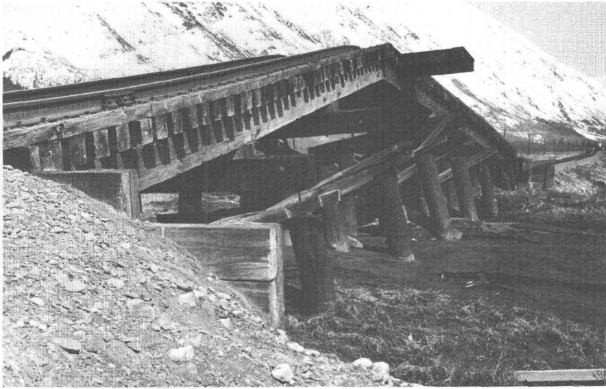
13.—Bridge 34.5 jackknifed upward by compression at the bulkheads. Note the mounds of fine-grained sediments ejected with ground water through cracks in the stream floor.
