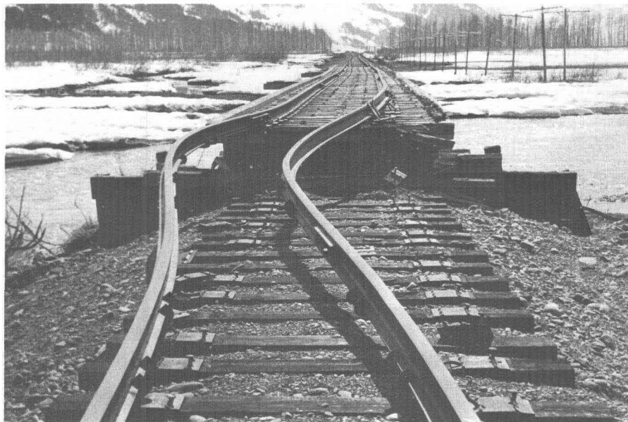
106.—View north over bridge 59.9 on Skookum Creek flood plain. It shows the lowered embankments, rails buckled by compression, and horizontal displacement of the embankment that produced a skew of about 3 feet in the bridge deck (see fig. 56).
