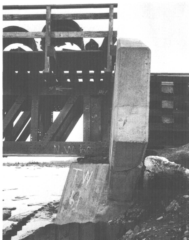
37.—Damage to Twentymile River bridge. Left: Concrete abutment broken away after earthquake to relieve pressure on spans. Note tilted bearing shoe and missing sheared-off anchor bolt. Right: North abutment backwall broken by thrust of steel deck.
