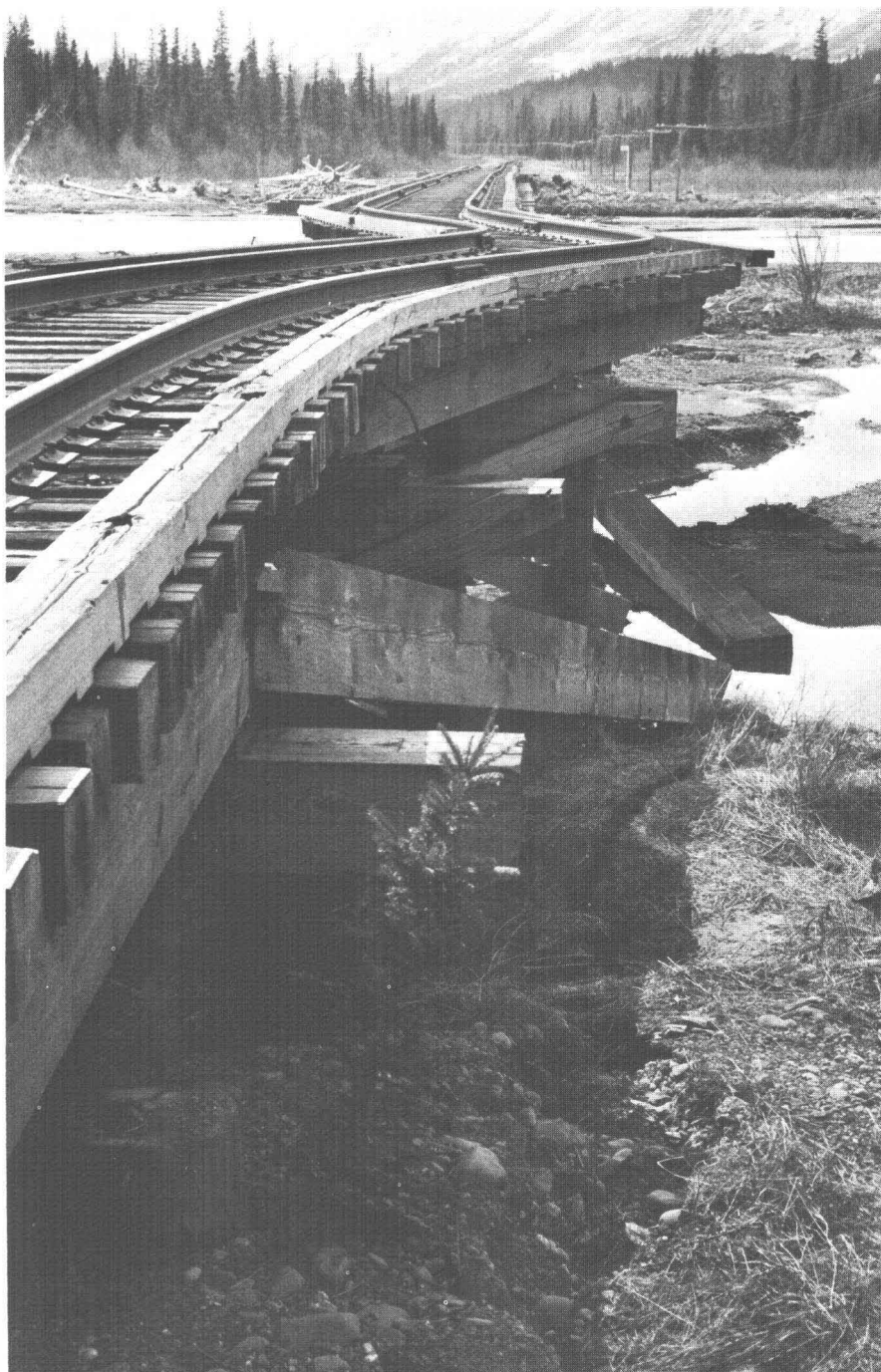
99.—Laterally buckled deck of bridge 37.0, on Hunter Flats. The buckling stringers broke free of some bents and pulled others (at apex of bend) laterally through the sediments.
