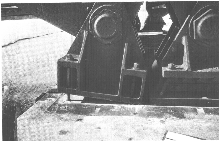
34.—Fixed end bearing lifted from pier at north end of sixth span of bridge 14.5. Anchor bolt pulled free of concrete. In adjacent expansion bearing, nested rollers were driven to the extreme position.
