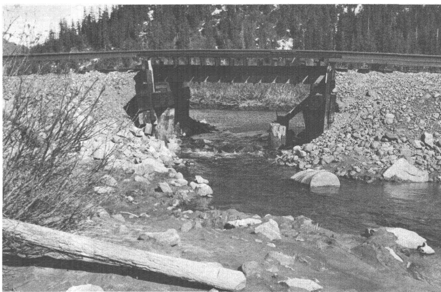
109.—View east at bridge 61.5 showing that the embankments were lowered relative to the bridge deck but had risen slightly toward the bridge.
