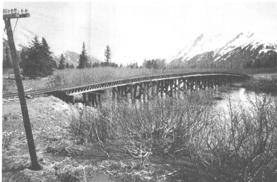
121.—A 2.6-foot arch in the deck of bridge 63.6 over Portage Creek. The deck was only slightly compressed, but was offset horizontally approximately 7 feet (see figs. 19, 56).
