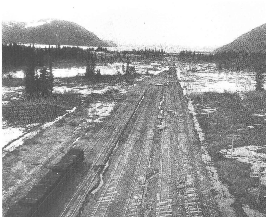
124.—Tension fractures between tracks on the Whittier branch marshaling yards. The subgrade fill failed by lateral spreading and the ballast failed in tension.
