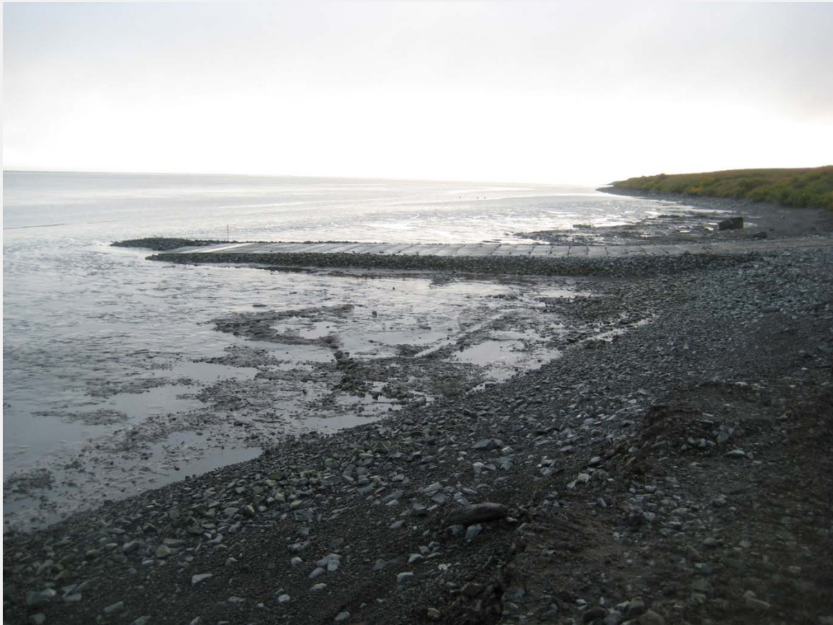
Figure 11: Mertarvik original barge ramp sinking in the mudflats. Photo taken in 2009 by R. Lundell, State of Alaska Department of Transportation.
