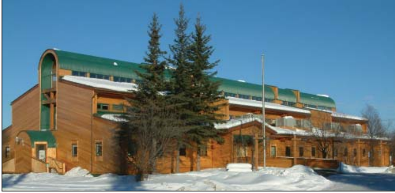
Division of Geological & Geophysical Surveys offices in Fairbanks
