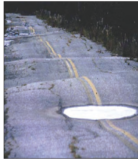
Figure 1. Thaw settlement of a paved bike path near Fairbanks, Alaska. Climate change may amplify thermokarst development as permafrost becomes warmer. Photo by State of Alaska Department of Transportation (DOT).
