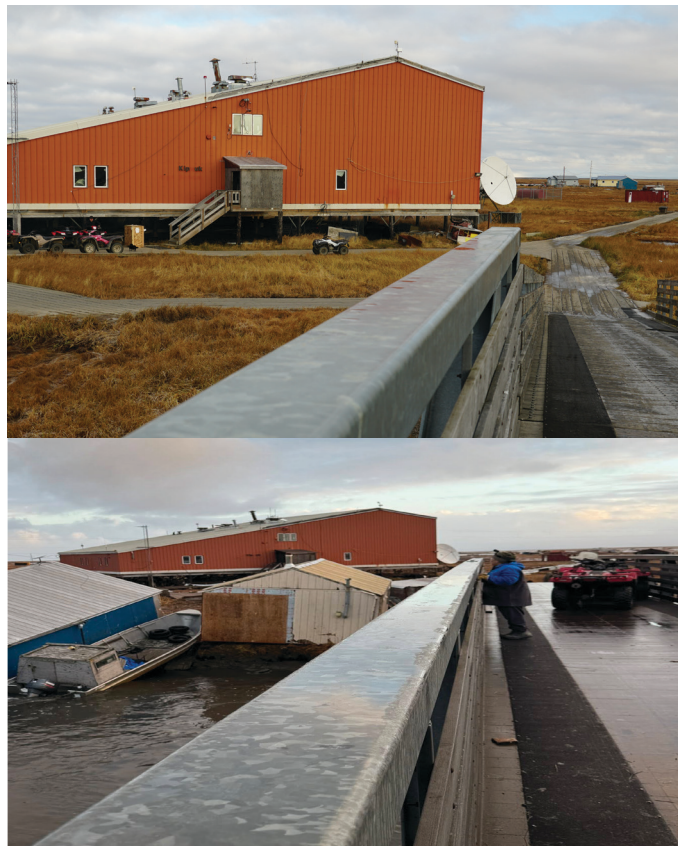
Comparison of bridge in Kipnuk, Alaska, before and after the October storm. Photo Above: Rayna Paul. Below: Nora Nieminski, DGGs.
