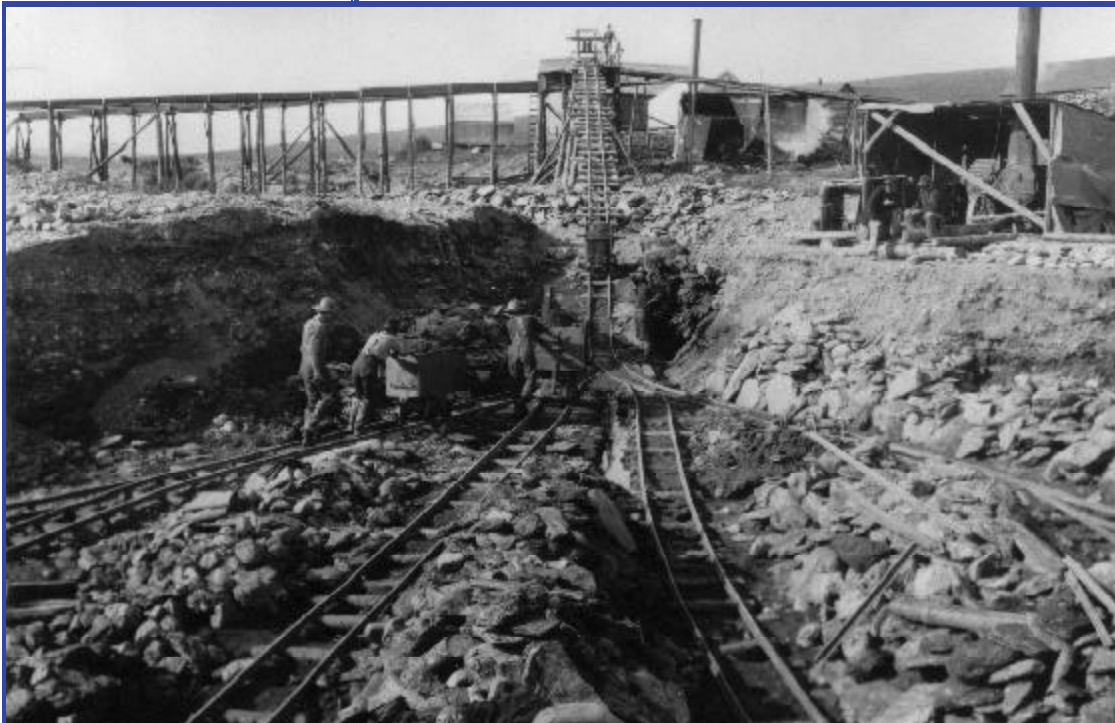
Incline hoist and pit at No. 15 Ophir, Wild Goose Mining Co., Seward Peninsula. VF Mining, Wild Goose, Accession no. 66-60-14, Archives, Alaska and Polar Regions Department, University of Alaska Fairbanks.
