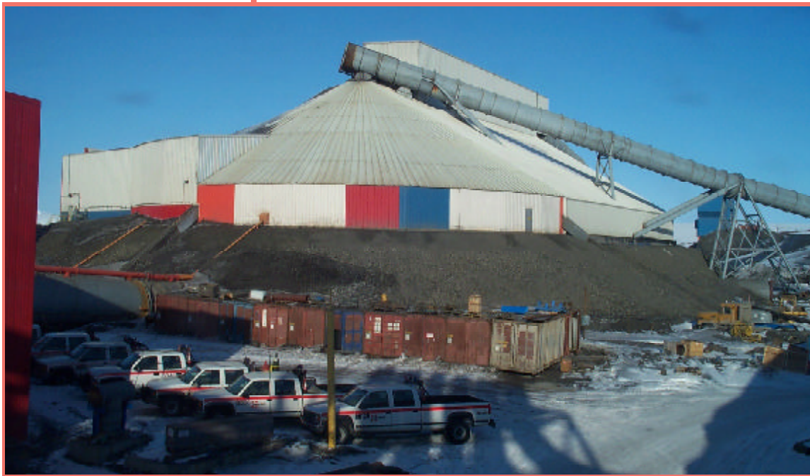
The “China Hut” ore haulage and storage facility at Teck Cominco’s Red Dog Mine in northwestern Alaska—the world’s largest zinc mine. Photo by D.J. Szumigala.
