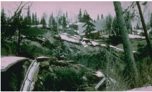
Landslide damage from the 1964 Great Alaska Earthquake.
