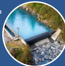
Power Creek. Credit: Cordova Electric Co-op
