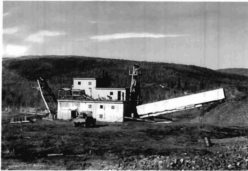
Fig. 1. Dredge operated by Minalaska, Inc. on upper Ganes Creek.
