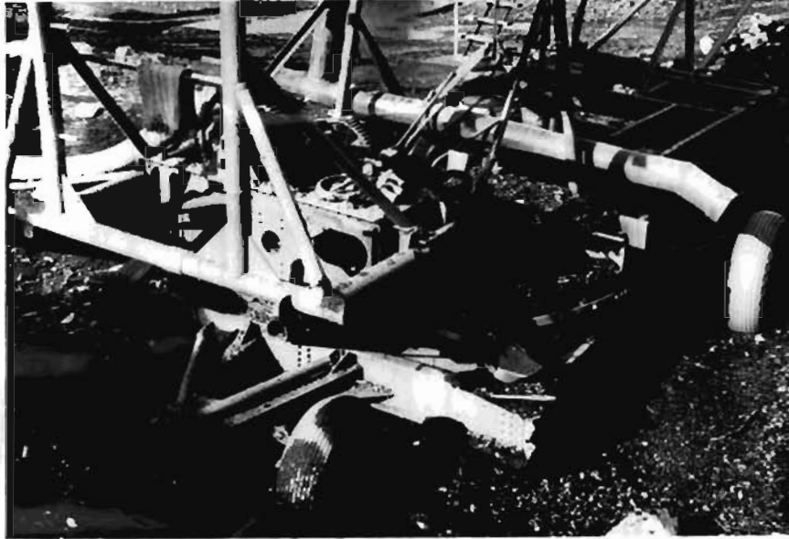
Fig. 6. Turntable base for sluiceway trestle, Flat Creek Placers.
