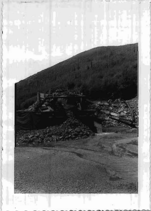
Fig. 7. Discharge end of Carstens' washing plant.
