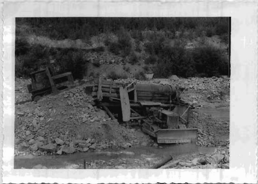
Fig. 6. Carstens' washing plant on Portage Creek.
