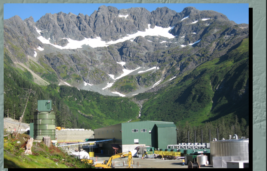
Mill, crusher, and processing plant at the Kensington Mine. Courtesy of Coeur Alaska, Inc. (Lode Mines ID-3)
