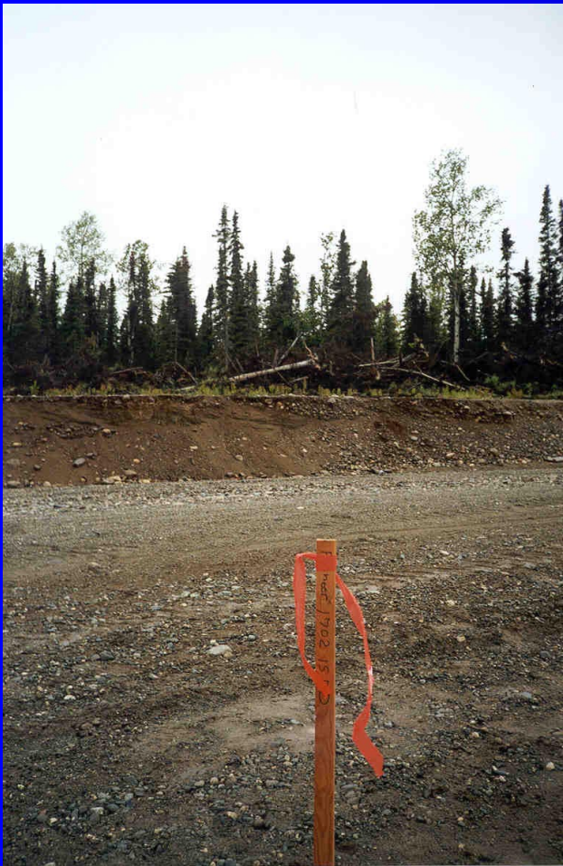
Pre- dirt Work
