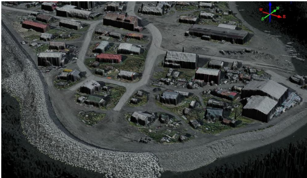
Figure 8. 3-dimensional model view of the Unalakleet revetment looking north from the inlet. (2014 aerial image draped over DEM provided by Fairbanks Fodar, 2014).
