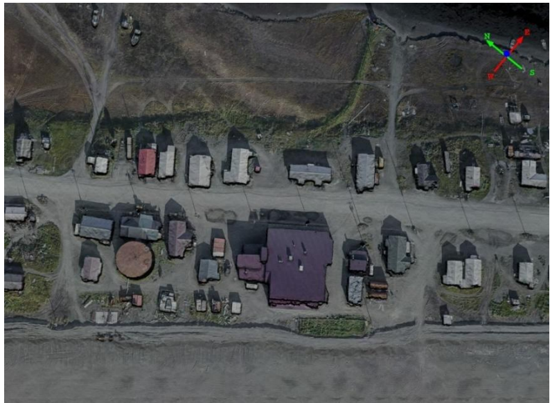
Figure 9. 3-dimensional model view of the berm project under construction in front of the Shaktoolik School (2014 aerial image draped over DEM provided by Fairbanks Fodar, 2014).
