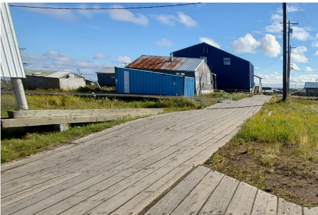
Figure 2. (Left) Photograph of a boardwalk affected by frost heave in Chefnak, Alaska. Photo: DGGS. (Right) Photograph of a home affected by thaw settlement in Tuntutuliak, Alaska. Photo: DGGS.
