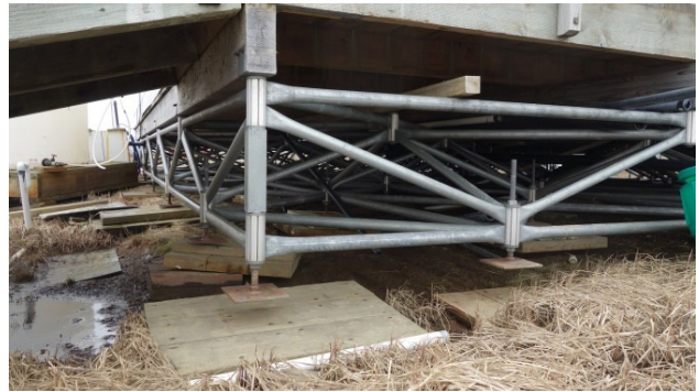
Figure 1. (Left) Photograph of local residents releveling a home in Kipnuk, Alaska. Photo: Golder Associates Inc.. (Right) Photograph of a structure's foundation footers affected by thaw settlement in Kipnuk, Alaska. Photo: AECOM.
