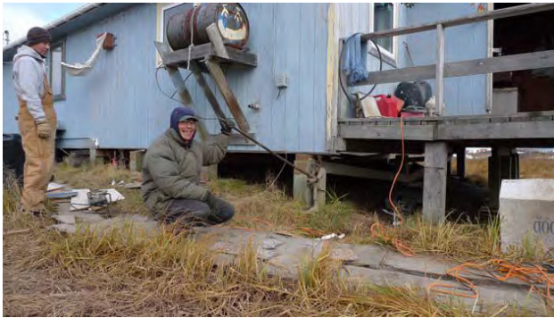
Figure 1. (Left) Photograph of local residents releveling a home in Kipnuk, Alaska. Photo: Golder Associates Inc.. (Right) Photograph of a structure's foundation footers affected by thaw settlement in Kipnuk, Alaska. Photo: AECOM.
