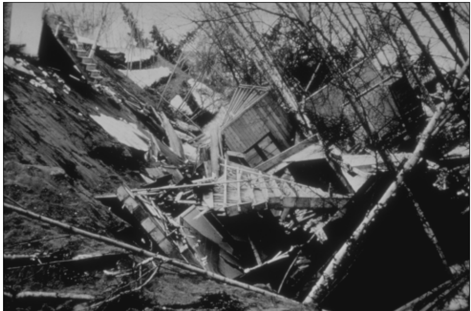
Figure 2. Damage in the Turnagain Heights subdivision of Anchorage in 1964, caused by earthquake-induced landsliding in an area underlain by weak, clay-rich soils. Photo from National Geophysical Data Center.
