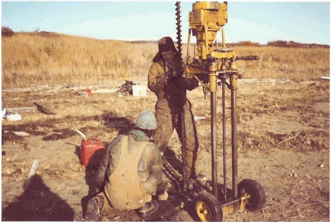
Figure 6 Drilling at Koyuk
