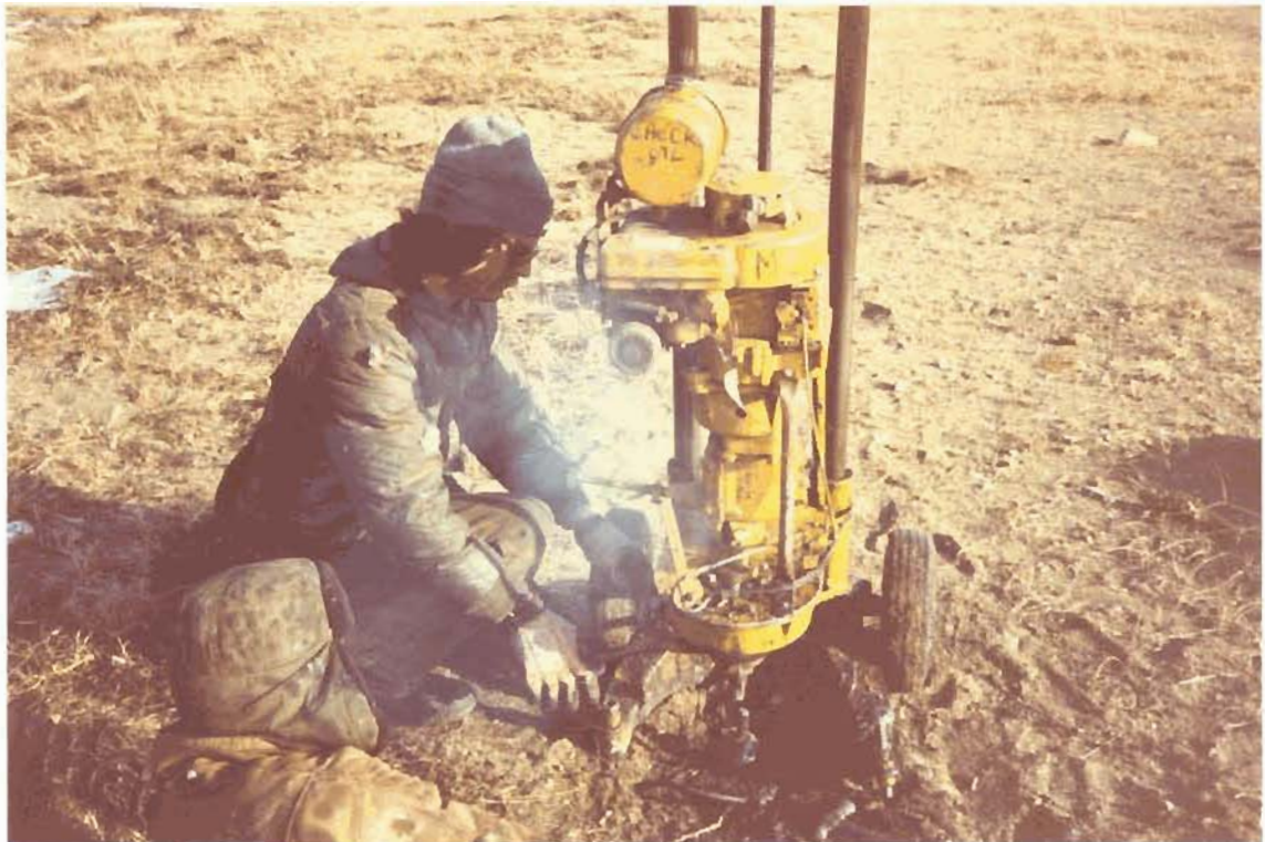
Figure 7 Drilling at Koyuk
