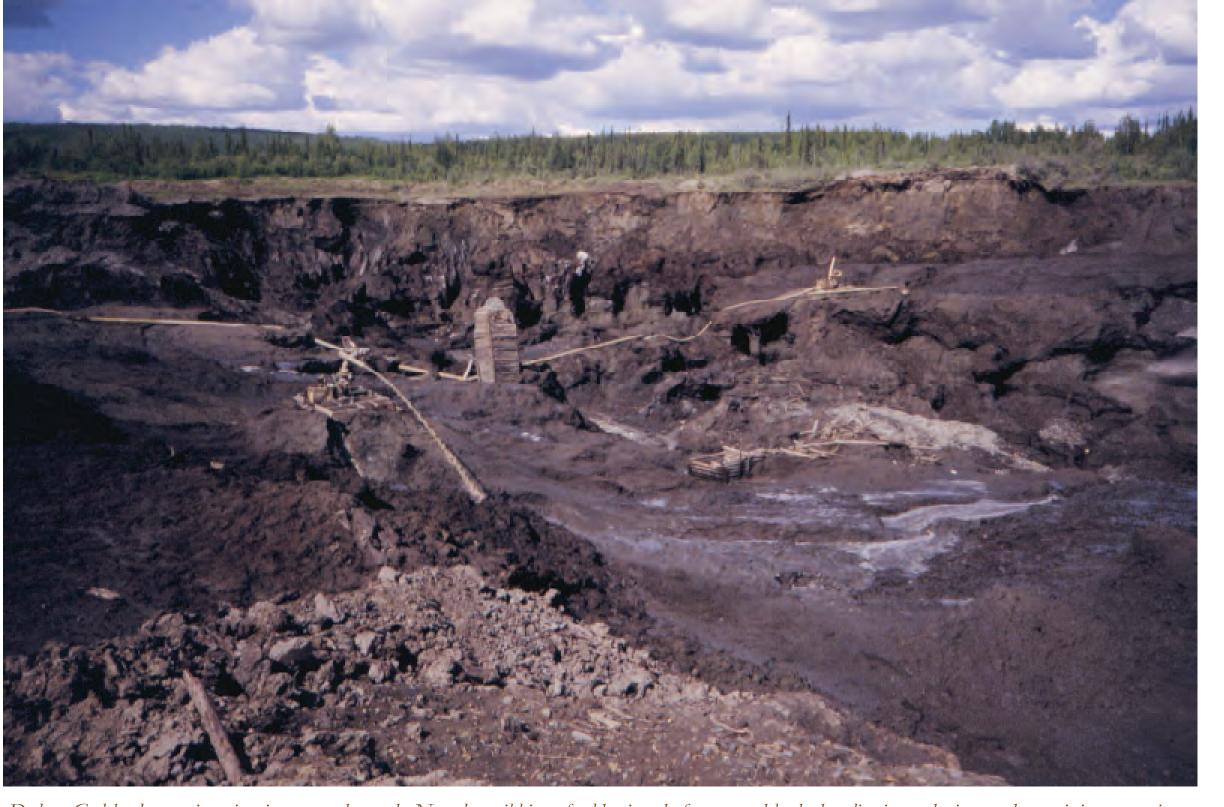
Dalton Gulch placer mine pit, view towards north. Note log cribbing of old mine shafts exposed by hydraulic giants during modern mining operations.
