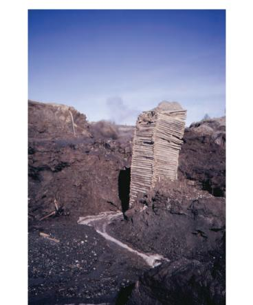
Mine shaft cribbing from early mining by ancient streamflow. operations exposed by hydraulic giants in Dalton Gulch.
