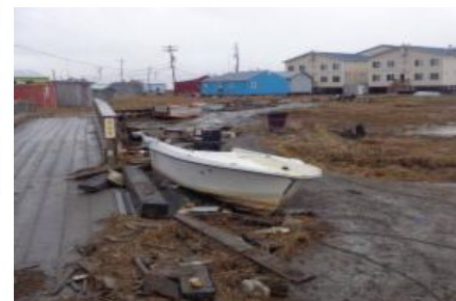
Kipnuk Storm Oct 28 2016 p06 Kipnuk EPA IGAP
