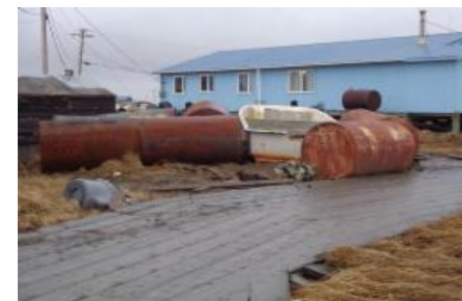
Kipnuk Storm Oct 28 2016 p03 Kipnuk EPA IGAP
