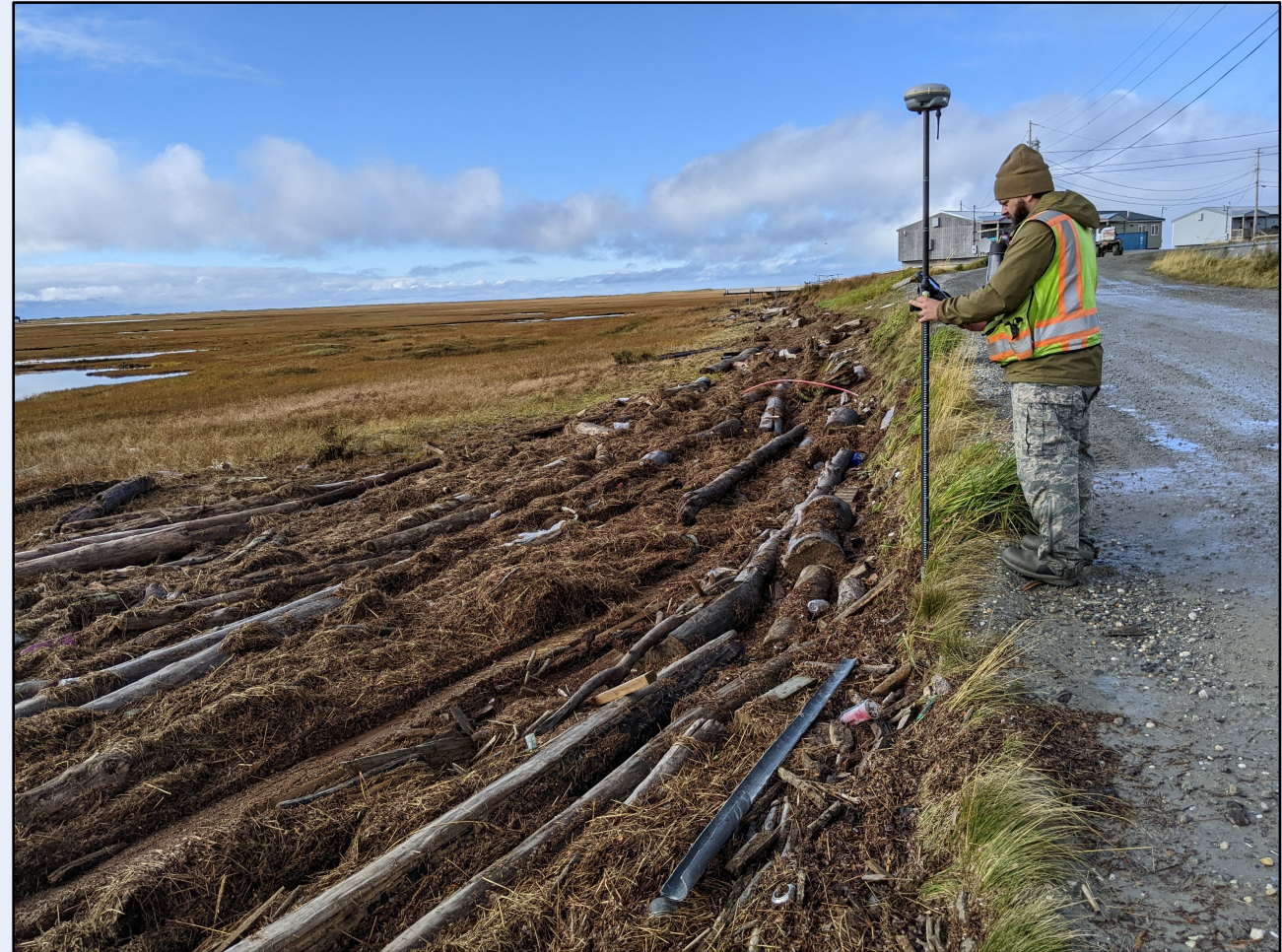
Ex-Typhoon Merbok debris line high-water mark in Hooper Bay, AK, on September 20, 2022
