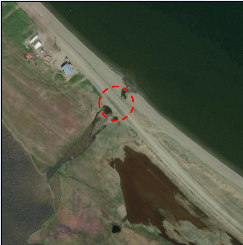
Culvert Assumed Clear
