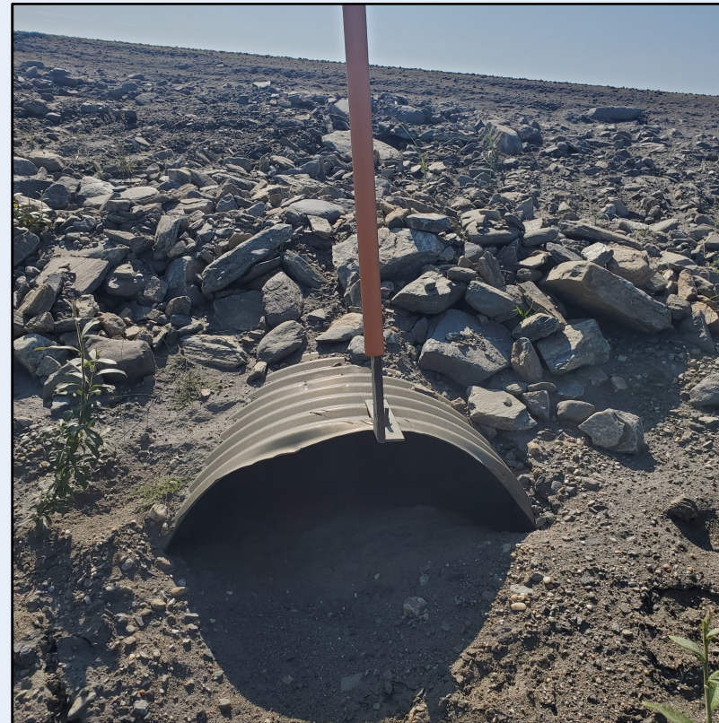
Culvert Blocked
