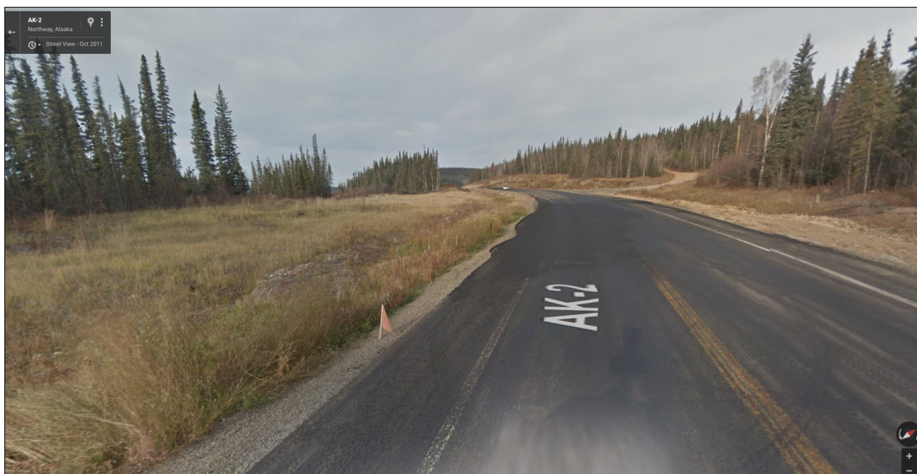
Figure 2. Google Earth Street View (October 2011) facing west-northwest along the Alaska Highway near milepost 1267. Notice the recently flagged and patched roadway in the east-bound lane; the first break in the tree line to the south of the roadway is the old, pre-2004 roadway.
