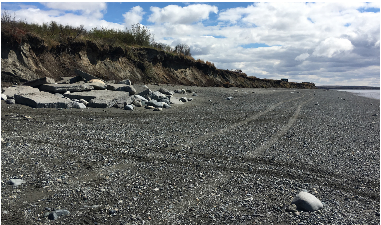
Figure 20. Erosion of coastal bluffs at Naknek. Photo taken May 2017.
