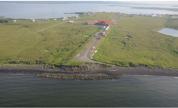
Figure 11. Oblique photograph of rock mound at St. Michael, taken July 2015 (ShoreZone, 2019).
