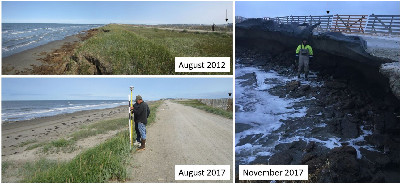
Figure 9. Erosion south of the rock revetments at Shishmaref between August 2012 and August 2017, as well as after a storm in November 2017 (photo provided by the Native Village of Shishmaref), with a stationary snow fence for spatial reference.
