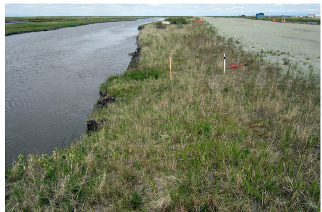
Figure 15. Erosion near the airstrip at Kwigillingok, which is also susceptible to permafrost degradation and flooding, which may lead to usteq. Photo taken June 2017.
