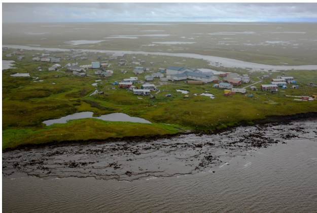
Figure 16. Oblique photograph of Newtok taken August 2014 (ShoreZone, 2019). Since then, erosion has begun to undermine the residential buildings nearest the river bank.
