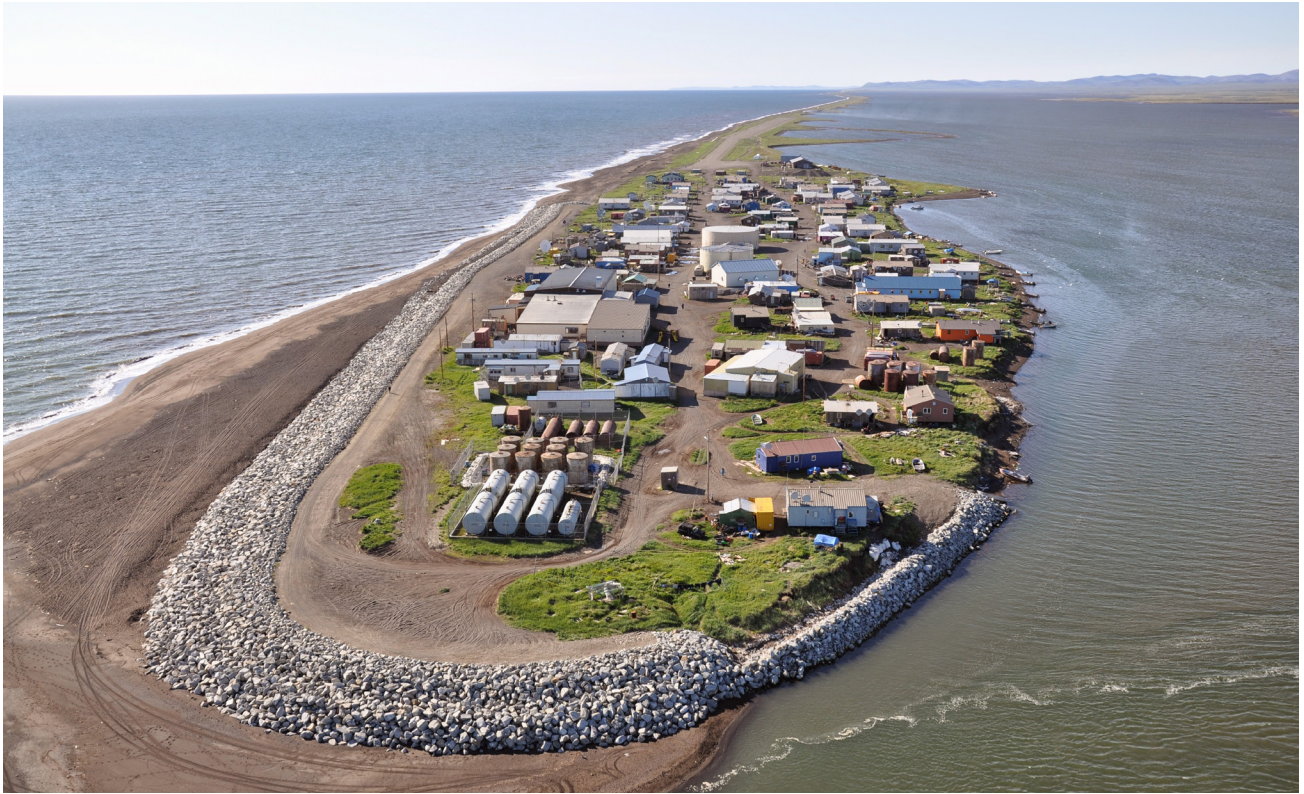
Figure 7. Oblique photograph of the rock revetment at Kivalina, taken July 2012 (ShoreZone, 2019).
