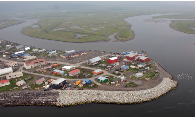
Figure 10. Oblique photograph of a portion of the rock revetment at Unalakleet, taken July 2015 (ShoreZone, 2019).
