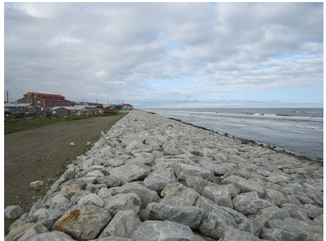
Figure 8. Shishmaref rock revetments. Photo taken August 2017.
