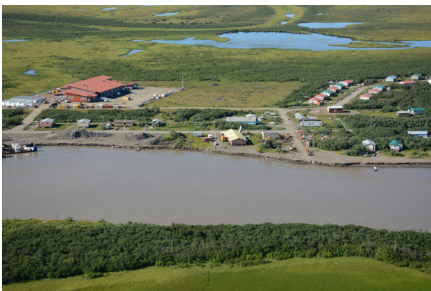
Figure 14. River bank at Alakanuk, where erosion has already undermined a road and other infrastructure. Photo taken August 2014 (ShoreZone, 2019).
