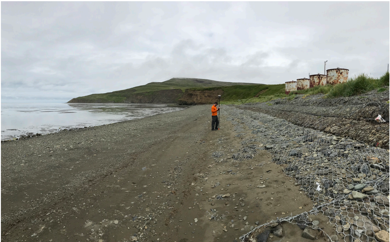
Figure 19. Gabion basket revetment at Tununak, August 2019.
