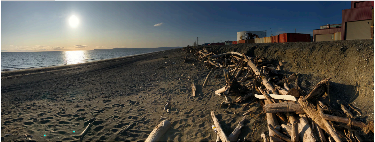
Figure 2. The eroded berm at Shaktoolik in front of the school and water tower after the August 2019 storm. The storm eroded much of the gravel, leaving the woody debris it was built upon.
