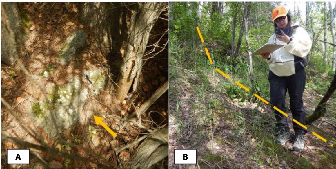
Figure A43. Images of BigB5_7S_6E_24_SE2 from July 1, 2020. A. Concrete near the toe, and (B) JAS standing along a slope break (indicated by dashed line) on the left flank. Photographs taken by MD.
