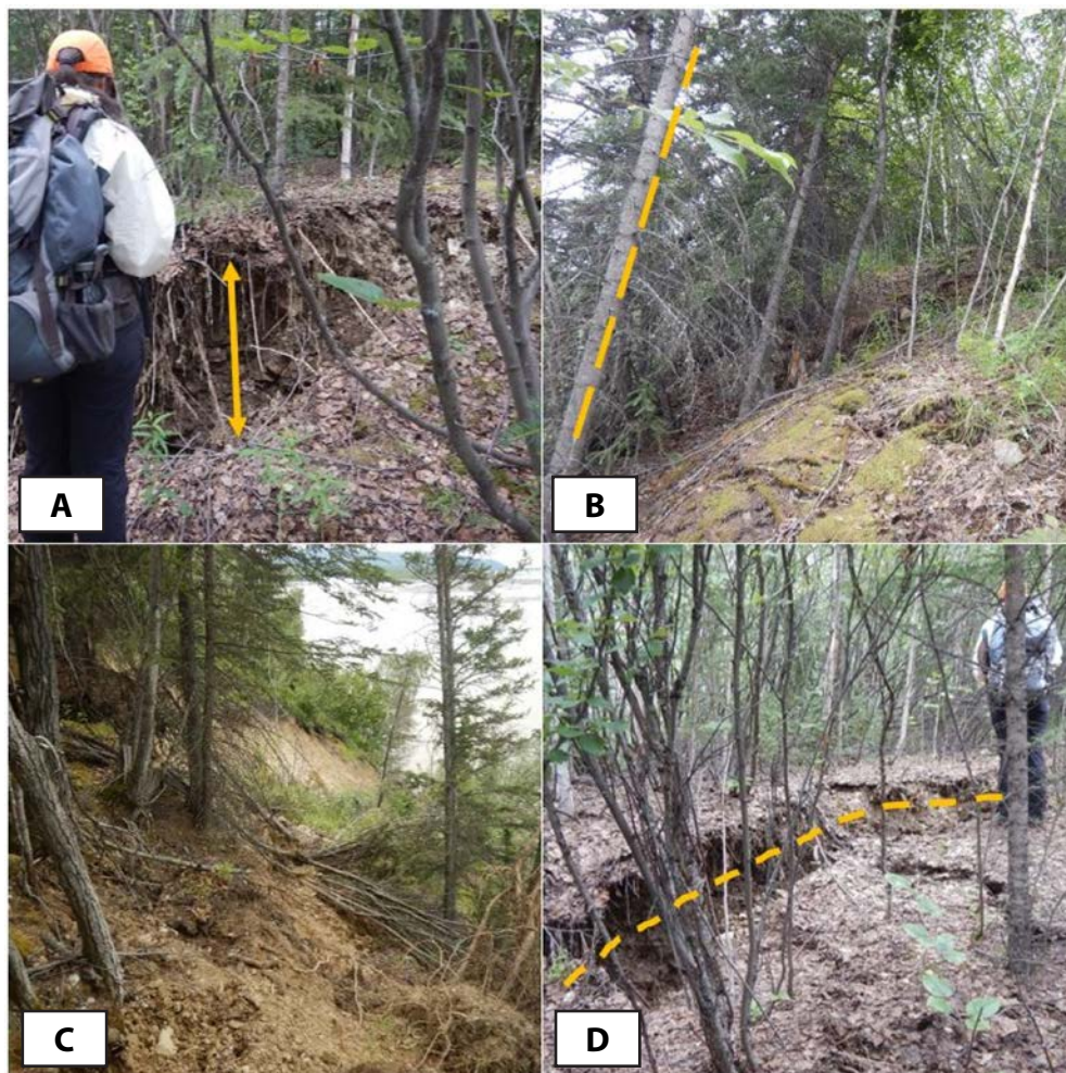
Figure A48. Images of BigB5_7S_7E_20_SW6 from July 2, 2020. A. JAS standing on a dropped block with a relatively fresh crack (arrows indicate separation), (B) cracks with leaning trees (dashed line indicates direction of lean), (C) head scarp with exposed soil near the river, and (D) JAS and a relatively fresh crack (dashed line positioned mid-crack). Photographs taken by MD.
