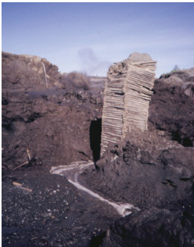
Figure 4. Log cribbing was used to reinforce shafts dug by early drift miners. Photo by D.S.P. Stevens, 1997.
